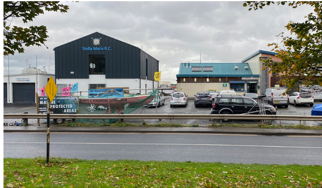
▲ View of existing boat clubs from a landscaped zone along the East Link Road, north of existing Great South Wall
