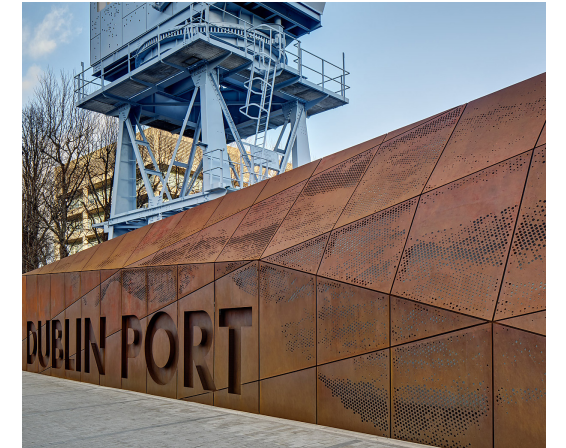
▲ Reference of sculptural corten wall at Port Centre, East Wall Road by Darmody Architecture
