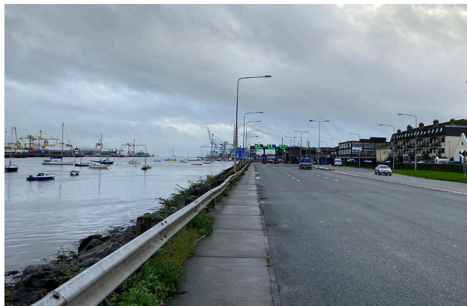
▲ Existing site condition along proposed ATR & Stop Point B facing east along southern revetment
