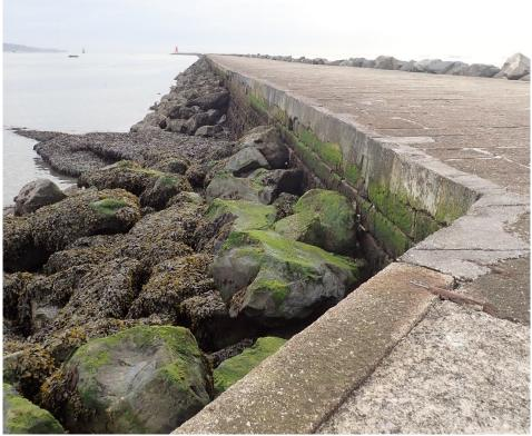
View looking east along GSW today just past White Bank Wharf Slipway ((DCIHR 19\_09\_011\_01). The rock armour protection placed at the base of the wall on the foreshore, and reaching the deck level on the south side are modern interventions
