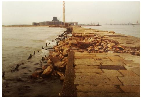
Photograph taken after the storm in 1981 shows damage to the GSW and a line of timbers off the south side, which appear to be the remains of 'The Piles'. Source: Dublin Port Company, Port Engineer
