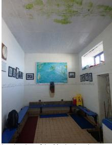
Interior view of the Men's changing rooms, showing blockwork interior and concrete roof
