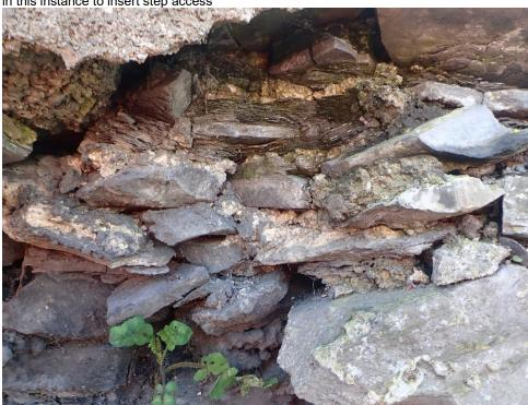
Detail showing fabric of the south parapet of the GSW in the MTL Yard where the wall core is exposed
