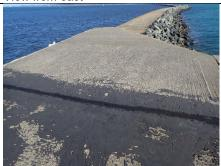
View looking west across the concrete roof of the bathing club, showing bitumen repairs
