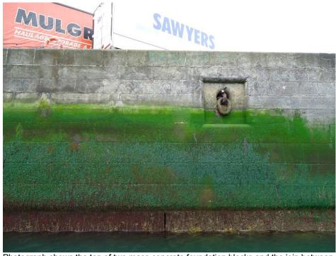
Photograph shows the top of two mass concrete foundation blocks and the join between both at the base of the image, with the granite ashlar coursing constructed above and a recessed mooring ring
