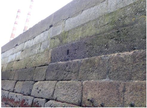
Detail view of north-facing elevation of harbour wall showing the stepped profile that it typical of the construction of the GSW.
