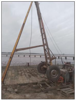
**Plate 11:** Cable percussion rig setup at BH-212 (Trench 7) on the landward side of GSW.
