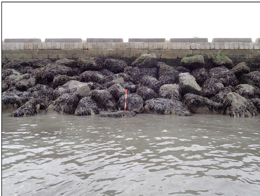
Plate 85: East-facing view GSW (north façade) showing extent of associated rock-armour protection, Survey Area 4, GSW-east (1m scale).
