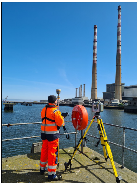
Plate 11: Laser-scan survey in progress at entrance to Pigeon House Harbour; scanning from the east dolphin of the Sludge Jetty.
