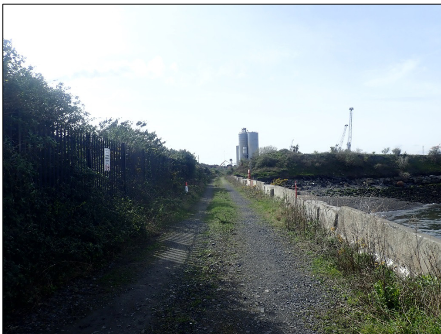
Plate 35: West-facing view along top of Feature F02; shot taken from west side of the entrance to the Sludge Jetty, note reclamation area in distance (1m scale).
