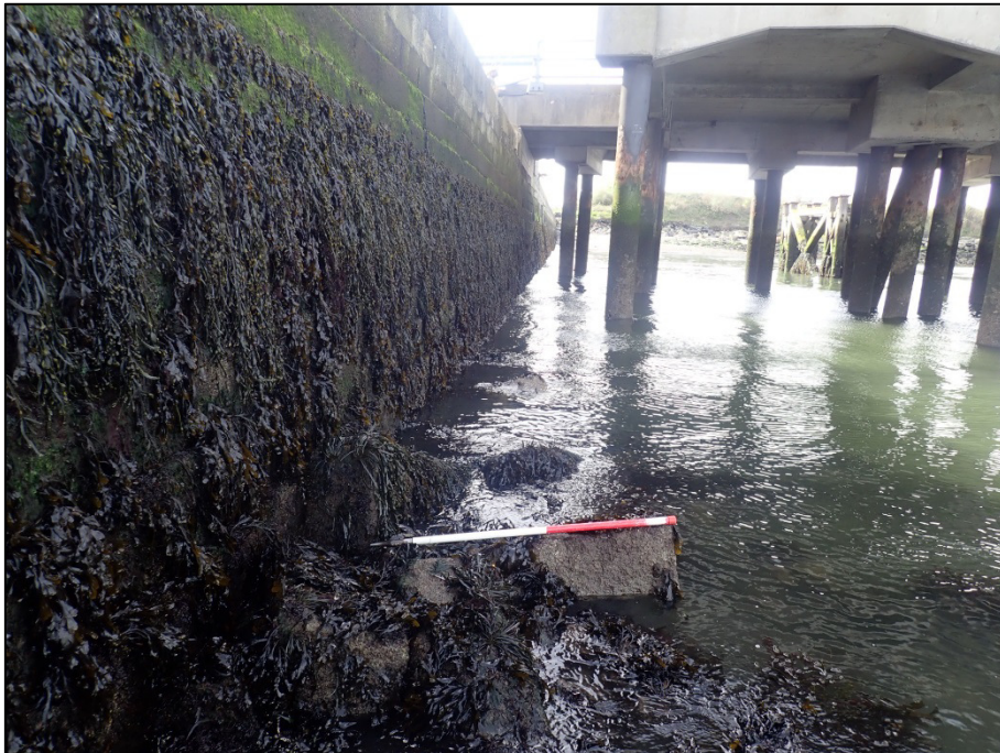
Plate 41: West-facing view along channel side of Feature F02, showing collapsed masonry from the pier-head access steps (RAS-02) in foreground and upstream Sludge Jetty in the background (1m scale).
