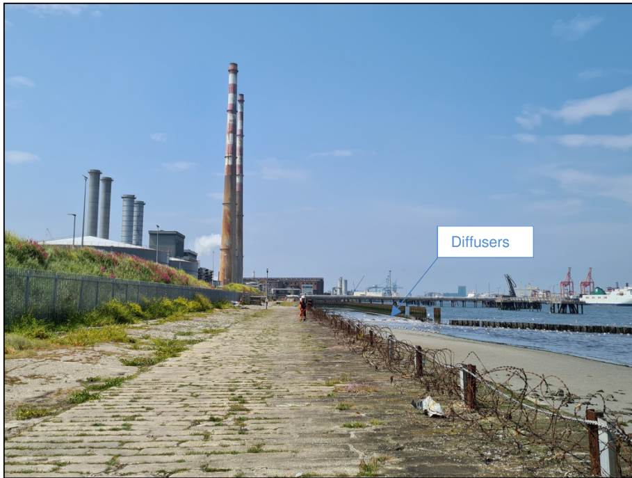
Plate 80: West-facing view along the surface of the sea-wall; Survey Area 4, GSW-east.
