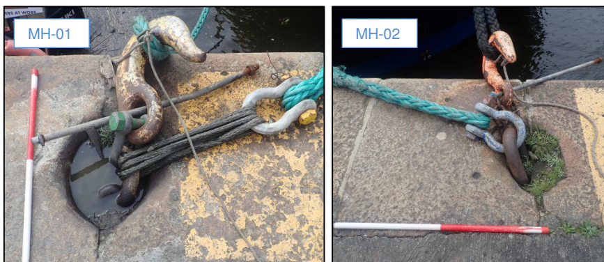
Plate 27: Two (2) sets of iron mooring-hoops (MH-01 and MH-02) which adorn the top of the NWQE at ITM 718048E, 734384N and ITM 718063E, 734382N (1m scale).
