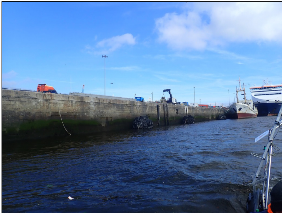
Plate 26: Northeast-facing view along NWQE, coming onto Low Water.
