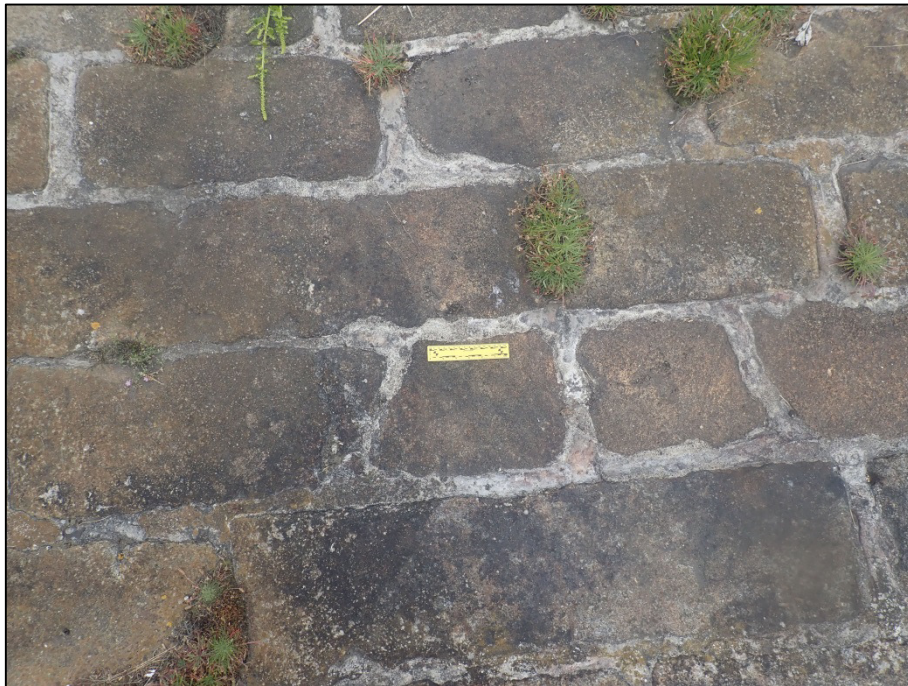
Plate 71: Example shot of deck masonry forming surface of the sea-wall (Survey Area 4, GSW-west 1); repointed using cement (150mm scale).
