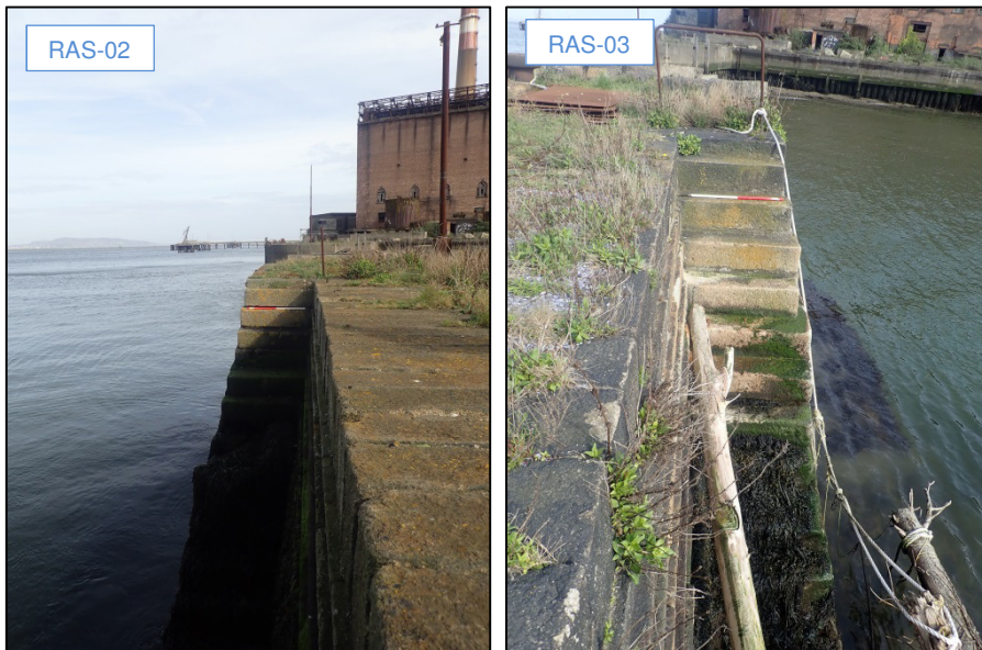
Plate 39: Opposing access steps, RAS-02 and RAS-03, located on the north and south sides of pier-head at the entrance to Pigeon House Harbour (1m scale).
