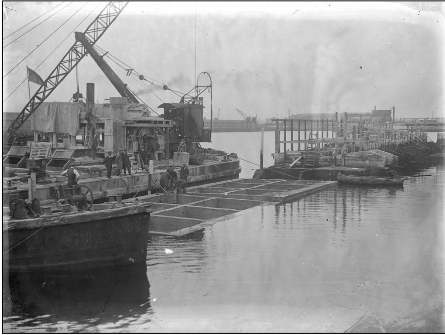
Plate 24: Early twentieth century photograph showing the use of floating caissons in the construction of new quaysides within Dublin Port [source: Dublin Port Archive].
