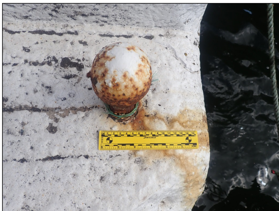
Plate 22: Detail shot showing well-preserved boat tie-off fitting from upstream river access steps; these being inset into every second step (150mm scale).
