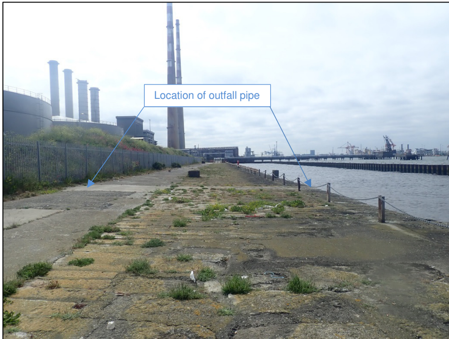
Plate 81: West-facing view of the surface of the GSW at the location of an outfall pipe that truncates the structure, Survey Area 4, GSW-east (1m scale).
