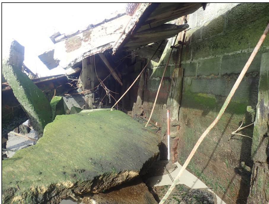
Plate 56: Original quay-wall (Feature F03) located behind the jumble of collapsed debris from a later quayside (1m scale).
