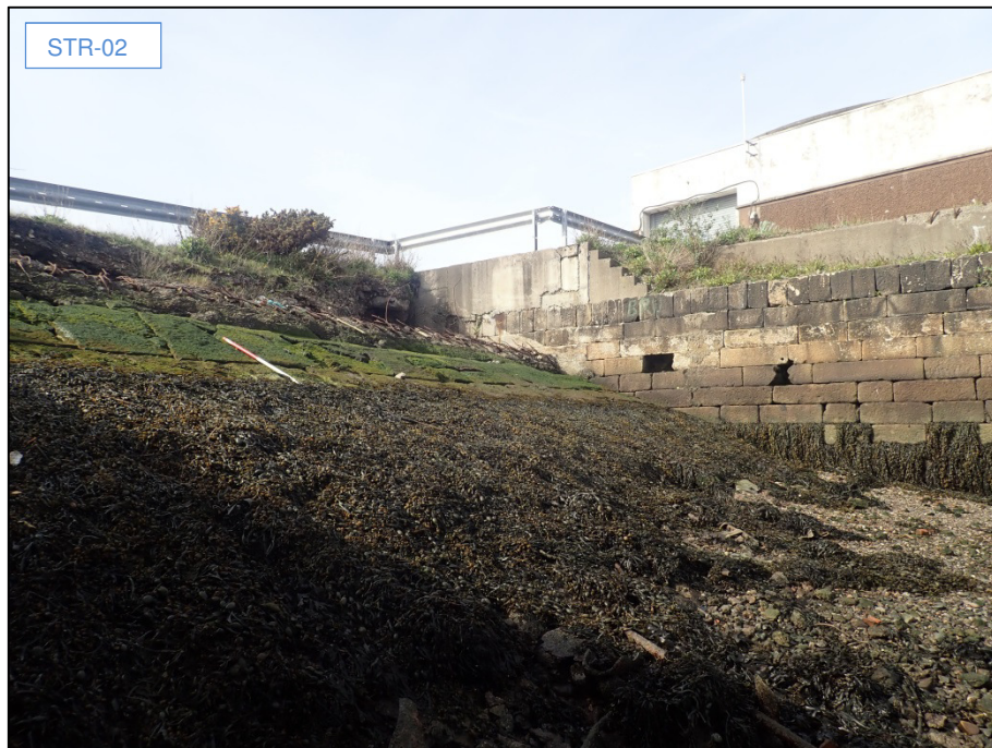
Plate 46: Northwest-facing view across face of angled retaining-wall STR-02 (1m scale).
