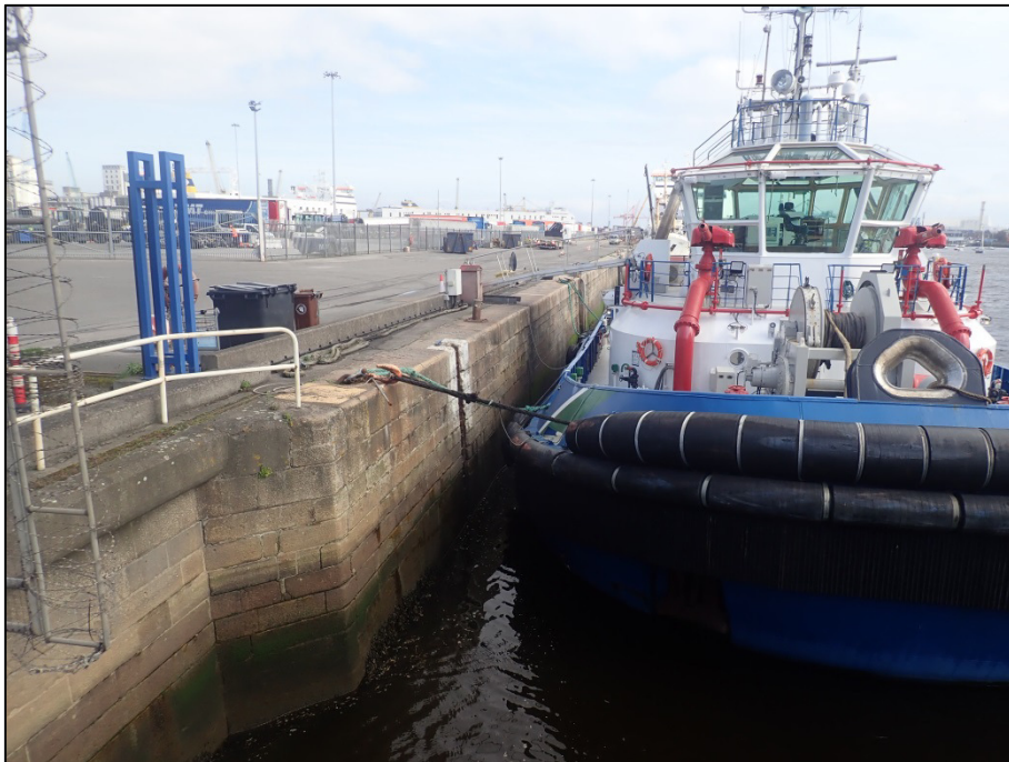
Plate 25: East-northeast facing view along NWQE, Berth 18.
