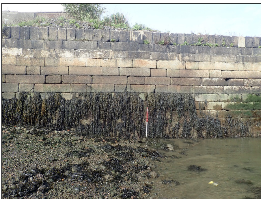
Plate 37: North-facing view of masonry comprising internal façade of pier-head, Feature F02 (1m scale).
