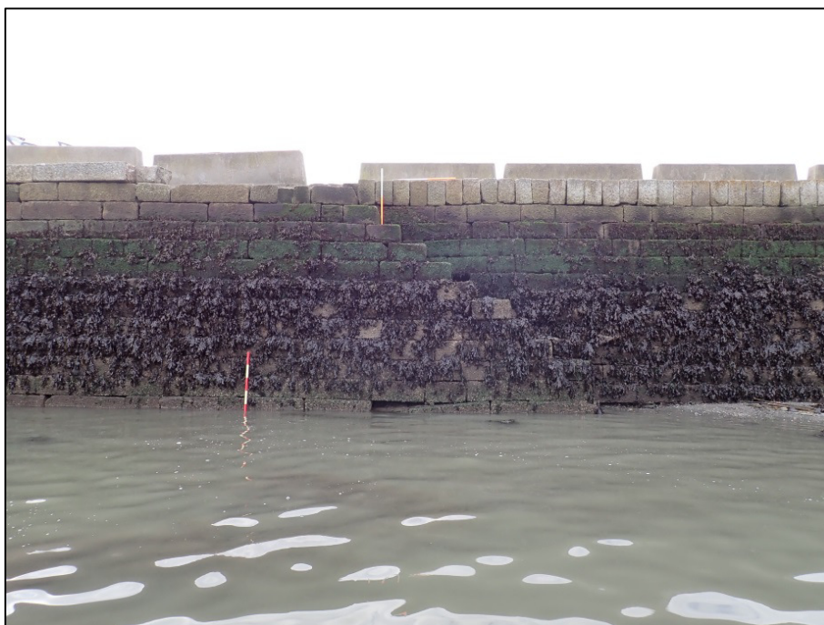
Plate 87: South-facing view of the GSW at location of set of masonry access steps, located short distance upstream of a boat-slip (STR-04); twelve (12) masonry courses visible for this section sea-wall (1m scale).
