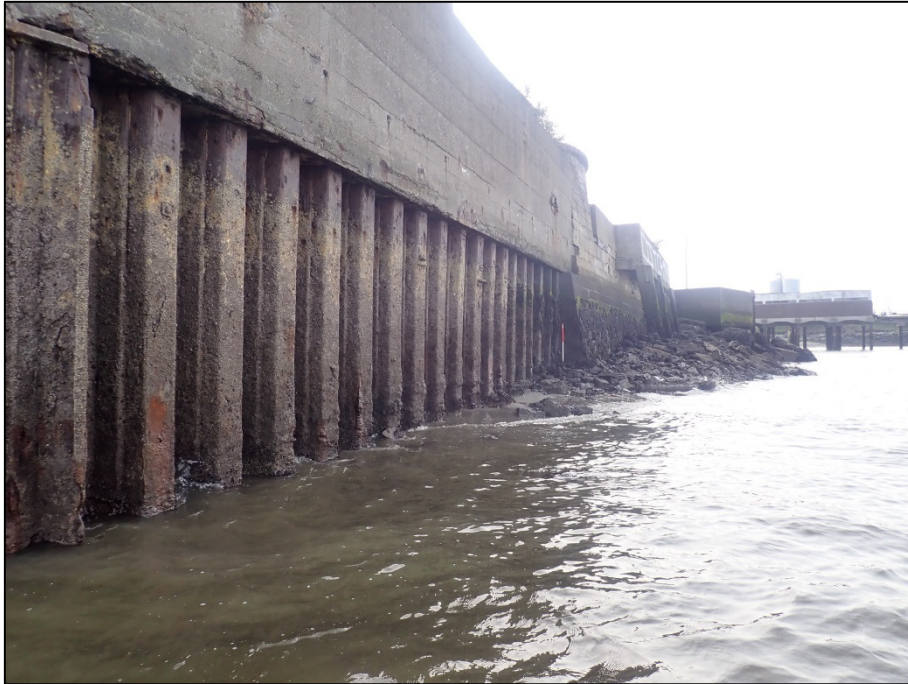
Plate 50: West-facing view along sheet-pile wall located to the east of a section of masonry façade comprising remains of Feature F02; east (1m scale).
