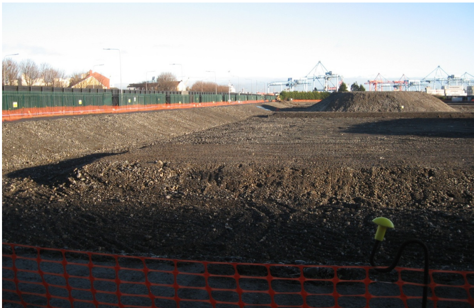
Photograph 2: site condition showing the perimeter berm
