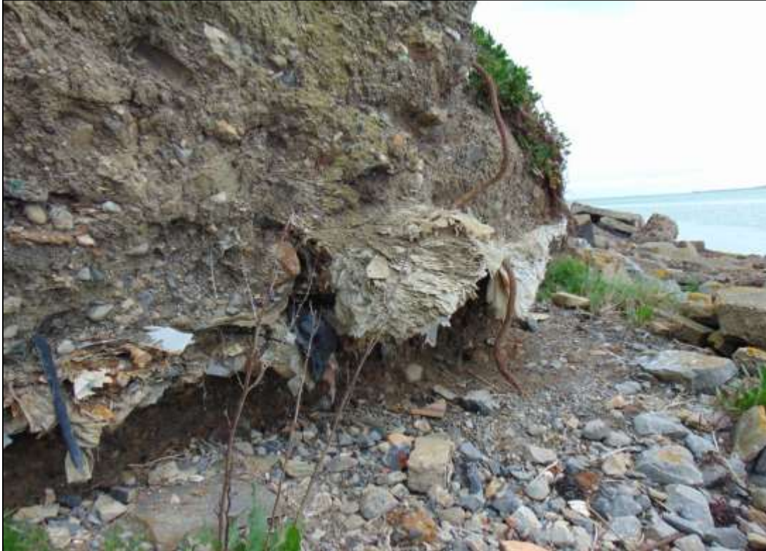
Plate 2-1: Waste exposure and signs of undercutting due to wave action
