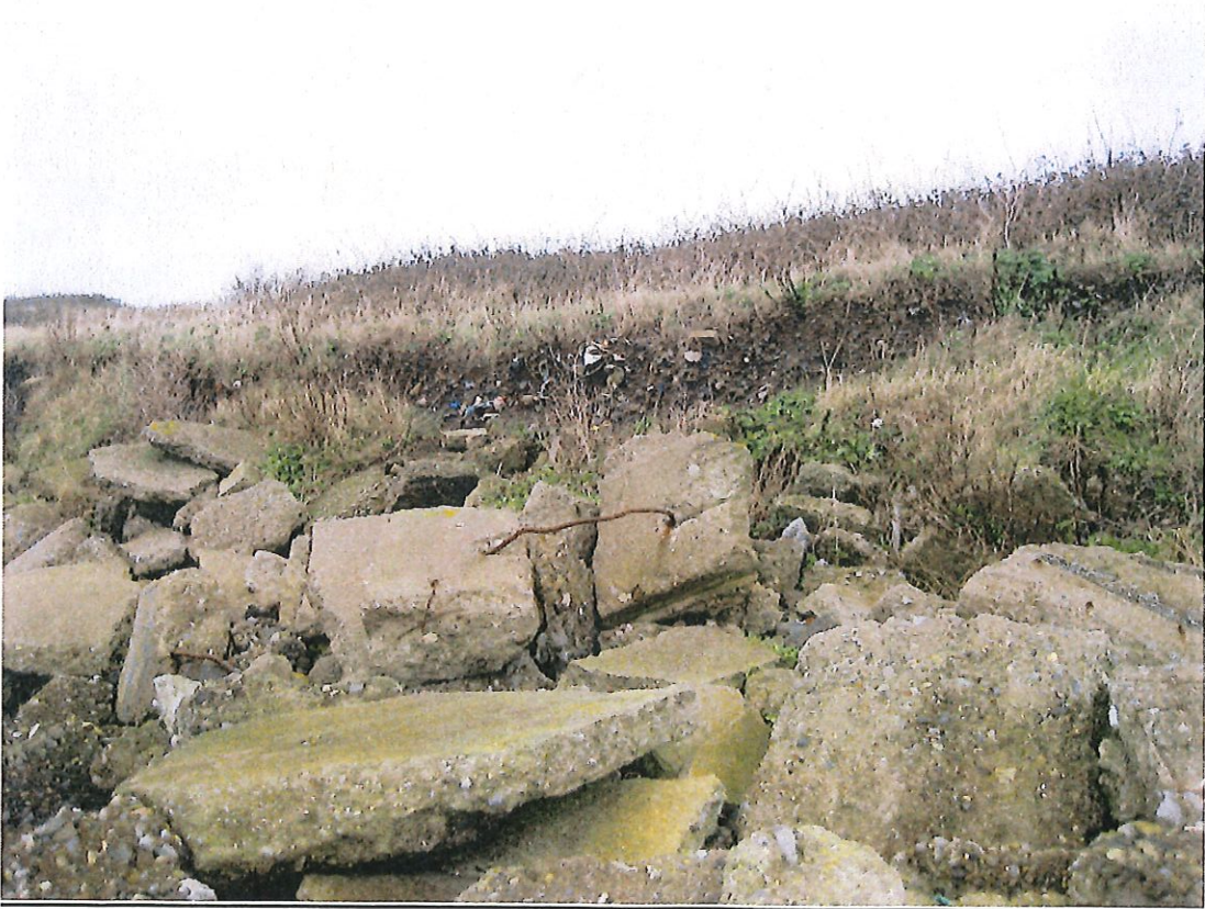
Photograph 4: Waste Exposed at Southern Face of Landfill
