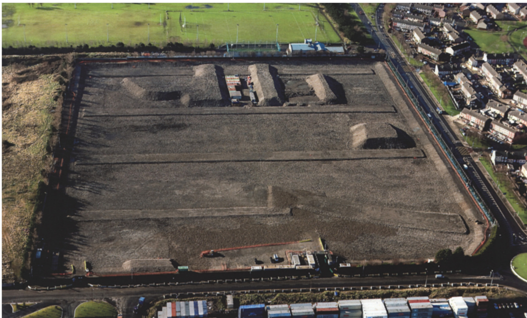
Photograph 3: Aerial photograph indicating the road footprints and stockpiles present
