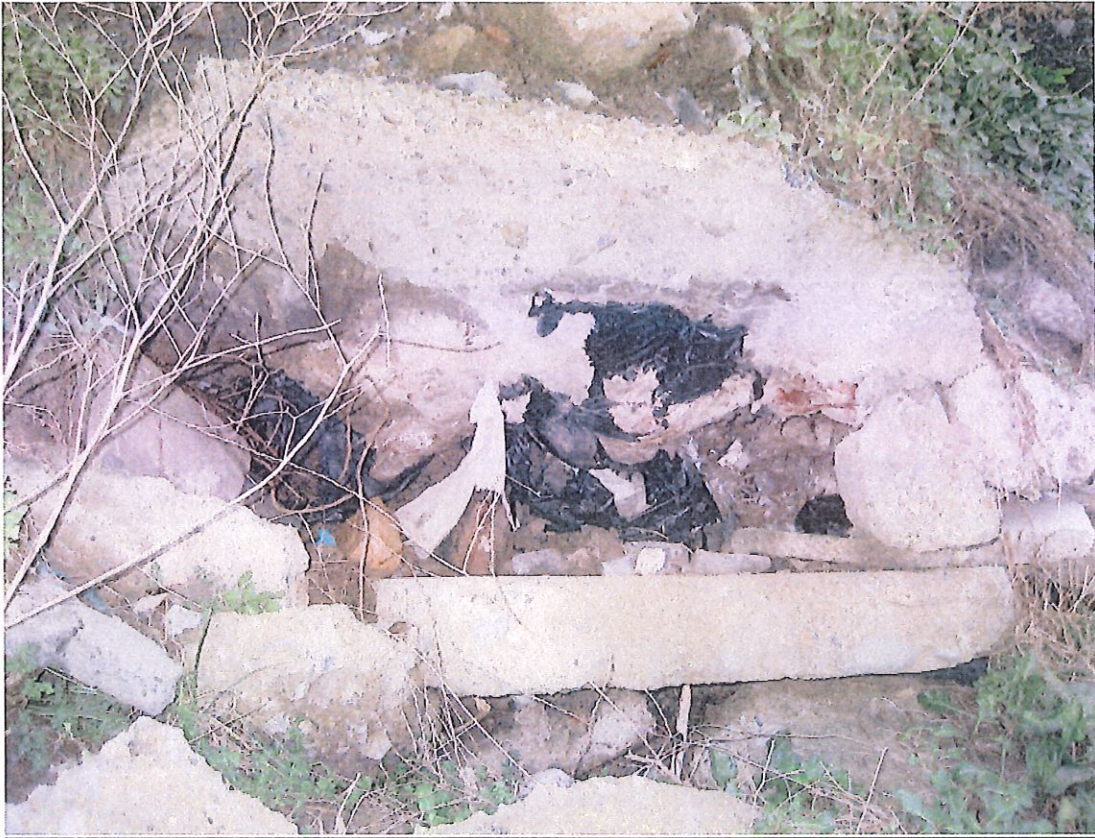
Photograph 8: Example of Waste Exposed
