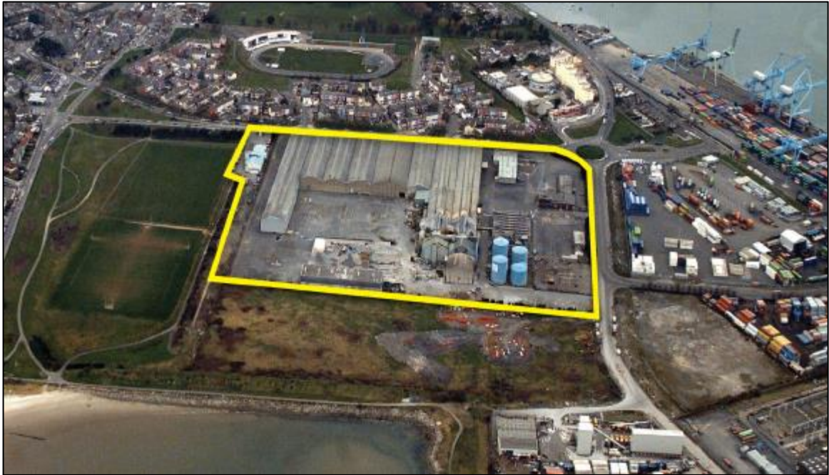
Figure 5-2 Aerial Photograph of the Irish Glass Bottle Site prior to remediation
