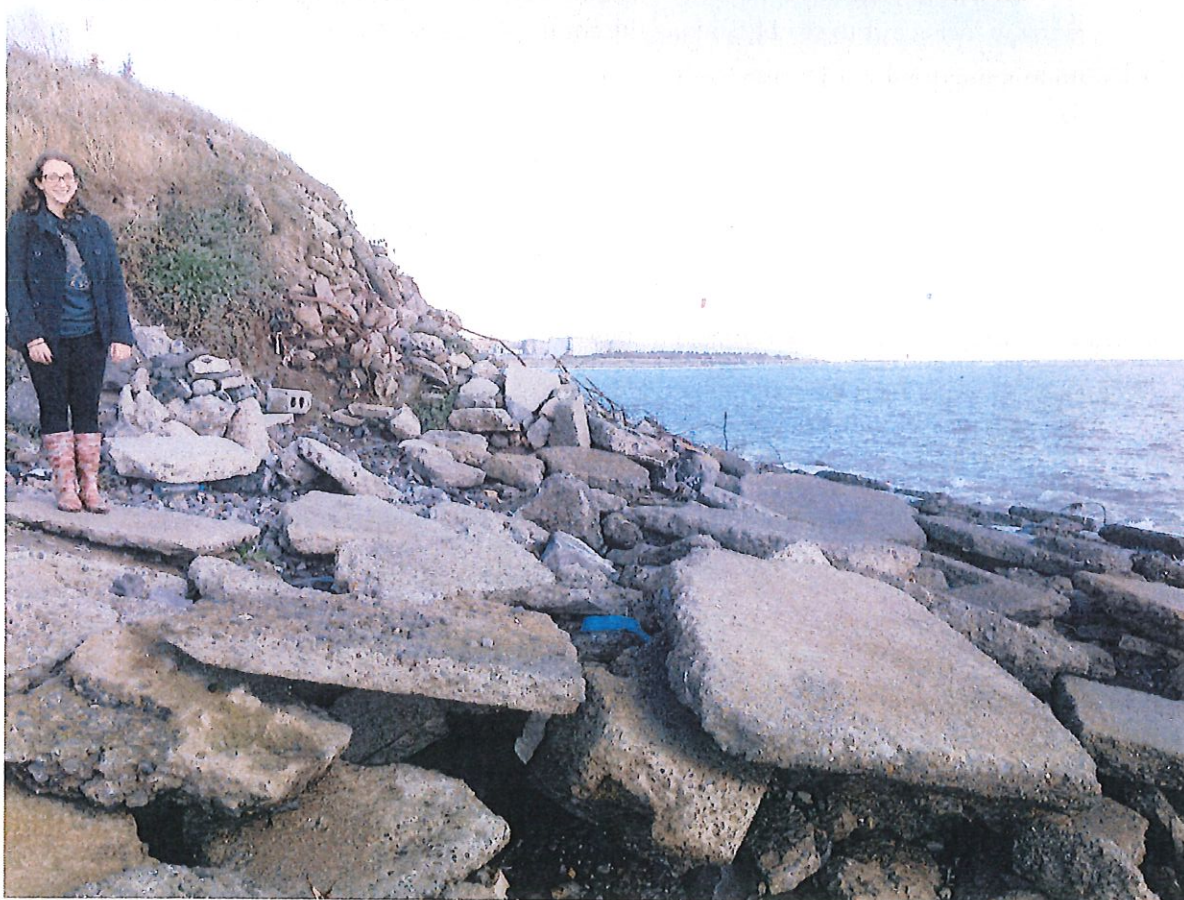
Image 3: High water line reaches well into the hard erosion control material of Ringsend landfill.
