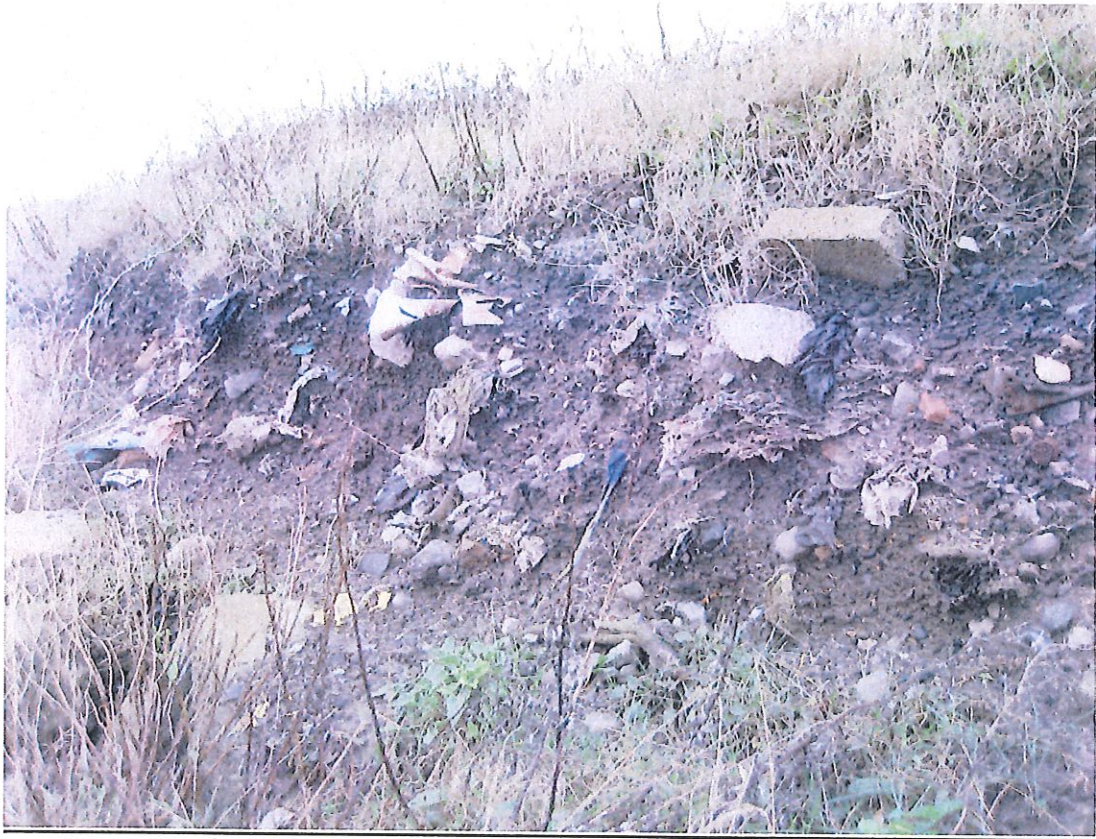
Photograph 7: Waste Exposed along Southern Face of landfill
