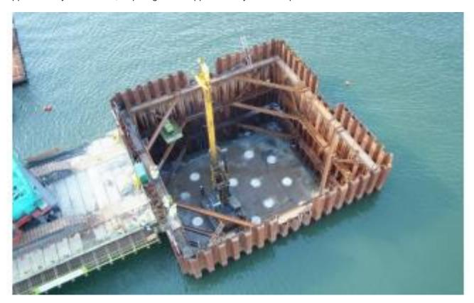
Figure 5.11 Example of cofferdam used during construction of Samuel Beckett Bridge.
