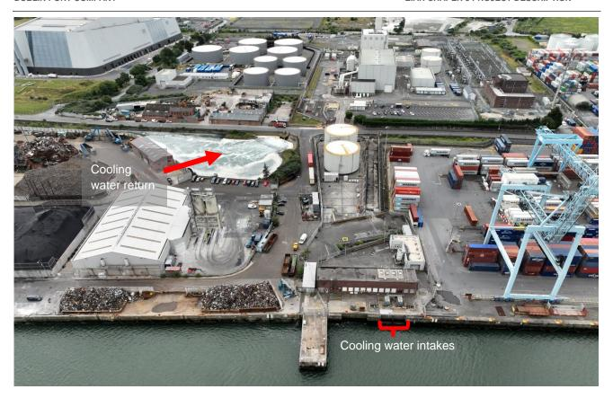
Plate 5.6 Synergen (Dublin Bay Power) Ringsend Generating Station from the north
