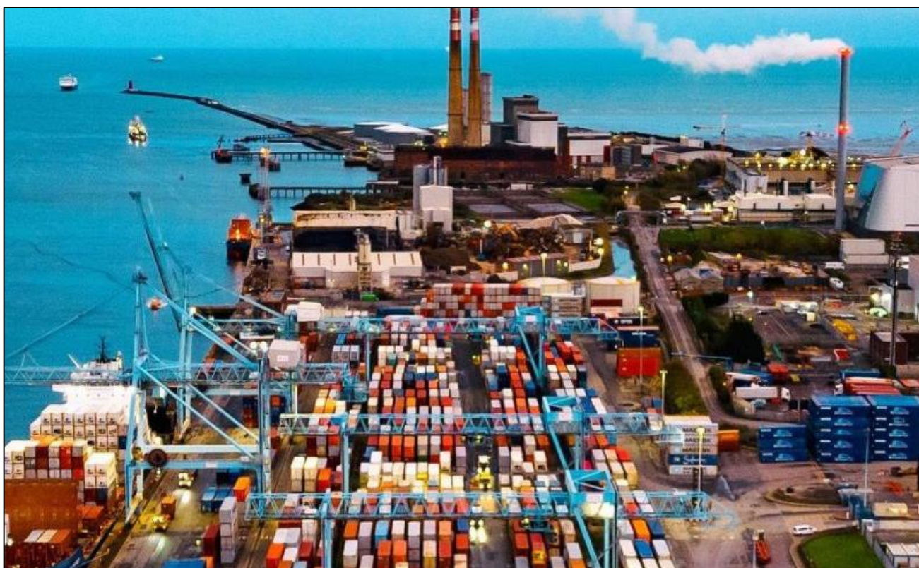
Plate 7.7 Typical hard standing within the development area
