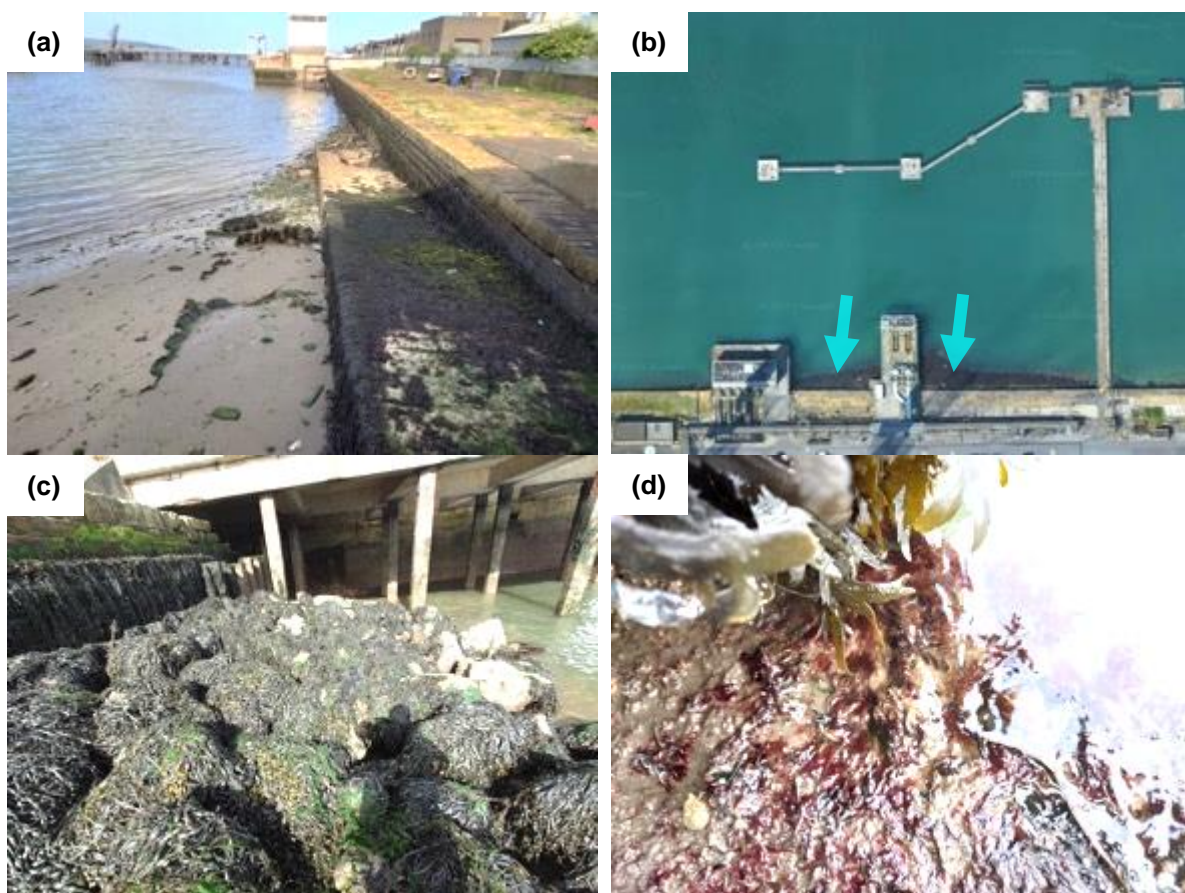
Figure 7.21(a) = the western end of the Great South Wall looking east toward the Poolbeg pumphouse and Oil Jetty. The southern boundary of the proposed new Area N Terminal will be kept 10m and 6m out from the Great South Wall which means that it will finish to the left of the furoid covered ‘slipway’ shown in Figure 7.23(a). (b) = a Google Earth aerial photo showing the two small areas of intertidal hard substrate just west of the jetty – (blue arrows). (c) = the top of the Great South Wall in the first of these boulder intertidal areas showing fine greens on top and Fucus spiralis below. (d) = general view of the shore toward the west showing the Ascophyllum covered boulders in the foreground and the shaded corner beneath the concrete platform on piles in the left background.
