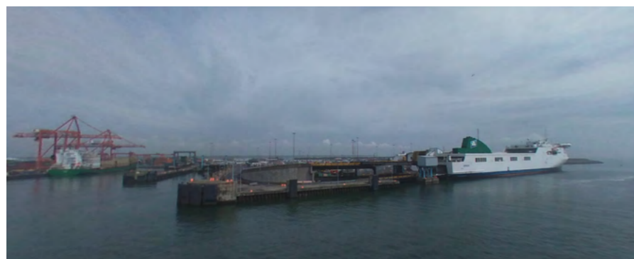
North Dublin Port reclaimed lands Source: Google Maps
