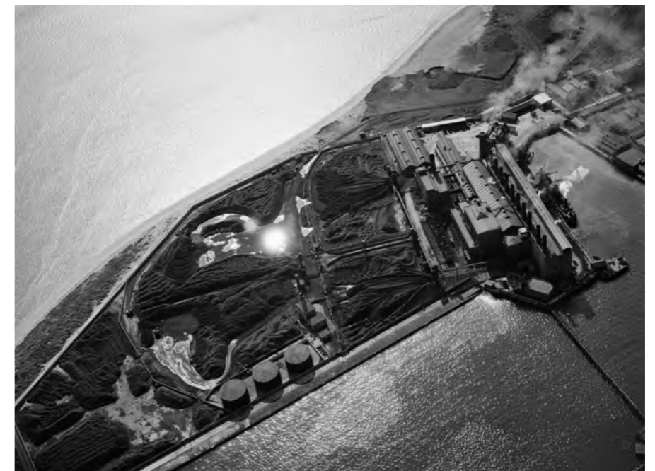
Pigeon House Harbour, view from above Source: Dublin Port Archive, ref 0519
