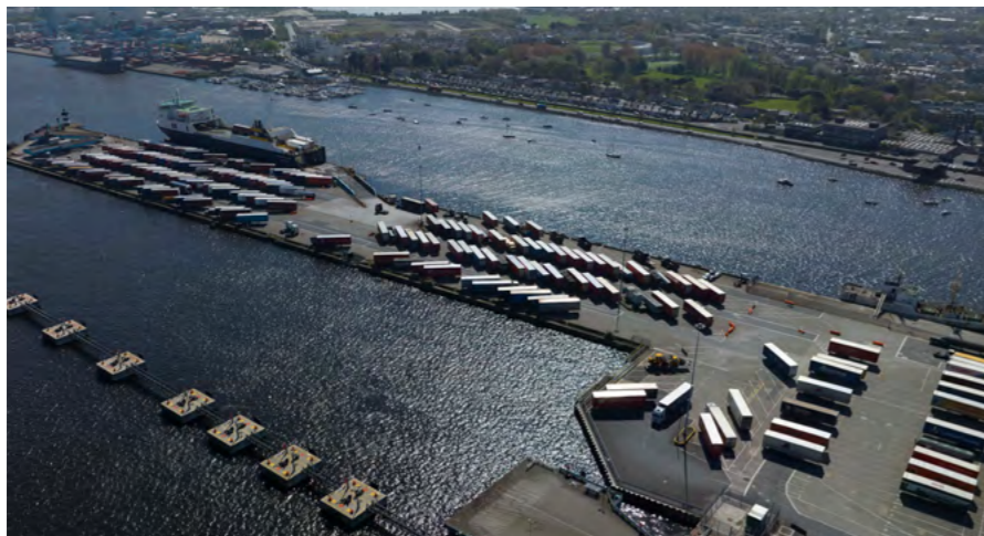
Alexandra Basin: Aerial view showing the new dolphin mooring, ramp and North Wall Quay Extension Source: Dublin Port Company Project Management Office
