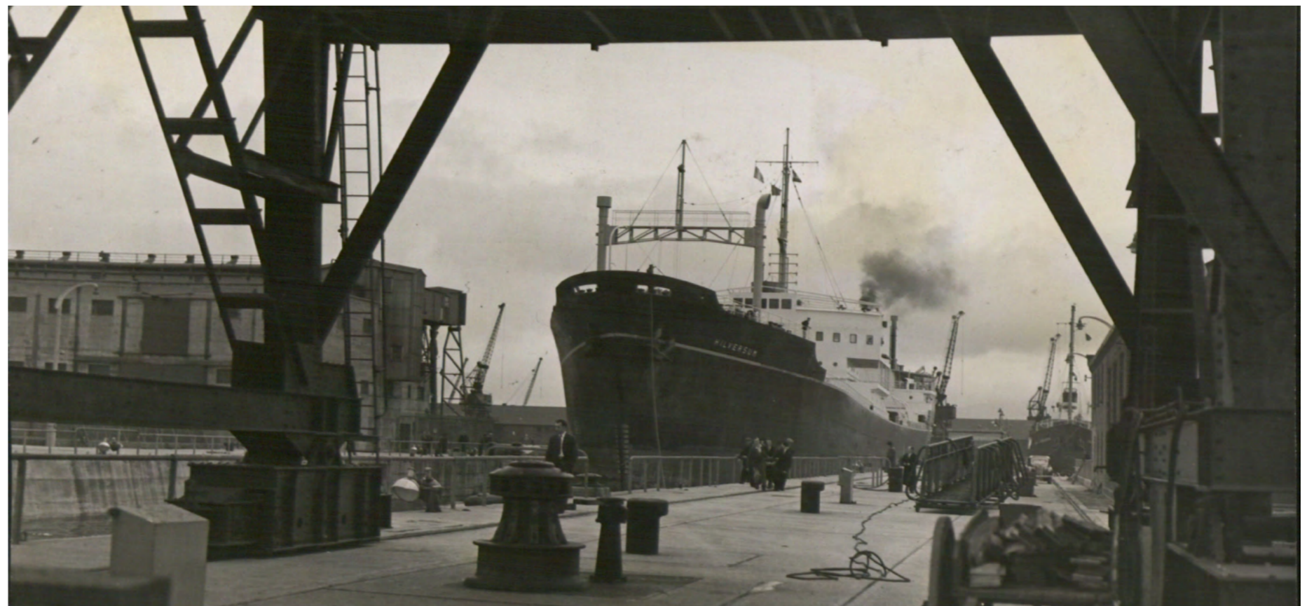
Hilversun at Graving Dock No. 2, 1959 Source: Dublin Port Archive
