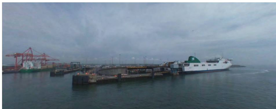
North Dublin Port reclaimed lands Source: Google Maps
