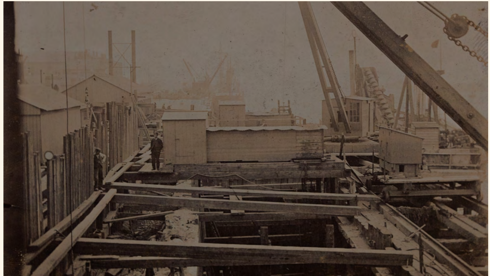
Historic photograph showing the construction associated with widening the quaysides in the nineteenth century. The specific location is not identified but it is likely to be along North Wall Quay Source: Dublin Port Archive, ref IMG 6068
