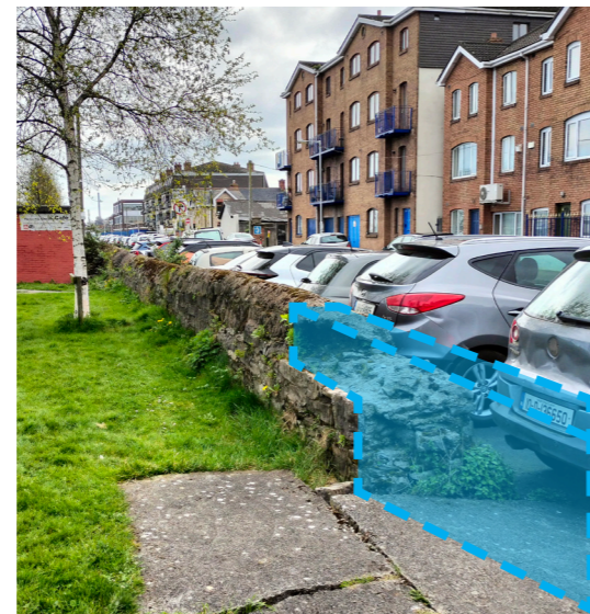
▲ 02. Section of the Great South Wall with segment removed for access route connecting public park and Fishermans Wharf residential.
