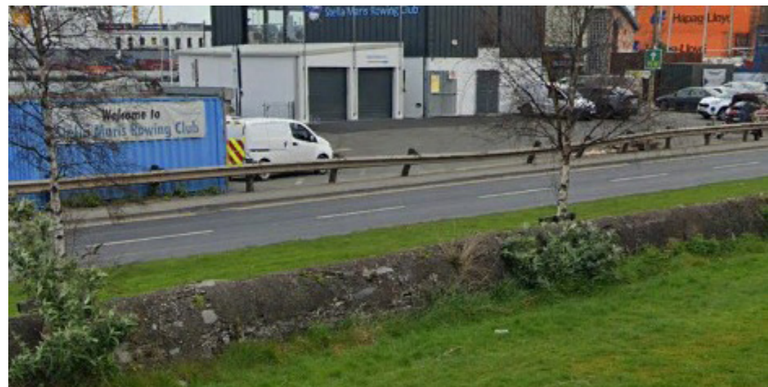
▲ 01. Section of the Great South Wall forming a boundary to Pigeon House Road and R131 adjacent to Stella Maris Rowing Club
