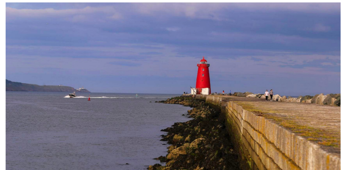
▼ 02. Section of the Great South Wall looking east towards Poolbeg Lighthouse
