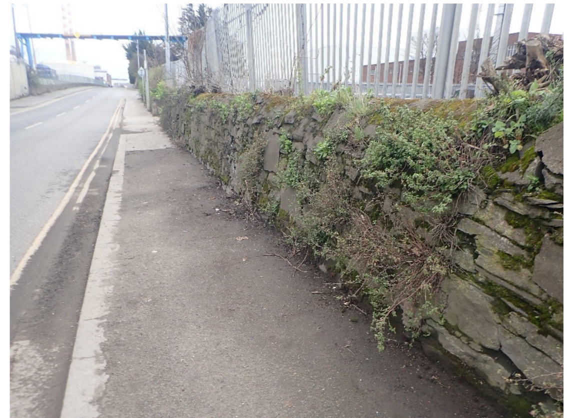
▲ Typical view of existing section of GSW in poor repair, courtesy of ADCO
