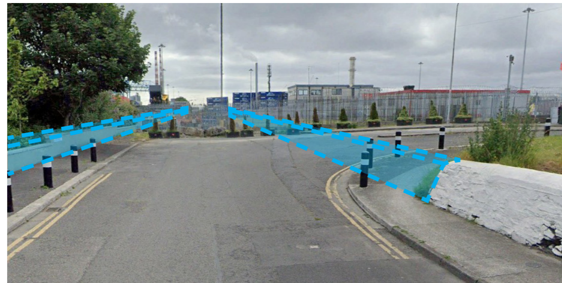
- - - Great South Wall Missing Portions
