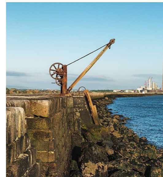
▲ 04. Section of the Great South Wall and cast iron crane looking west towards Poolbeg Powerstation
