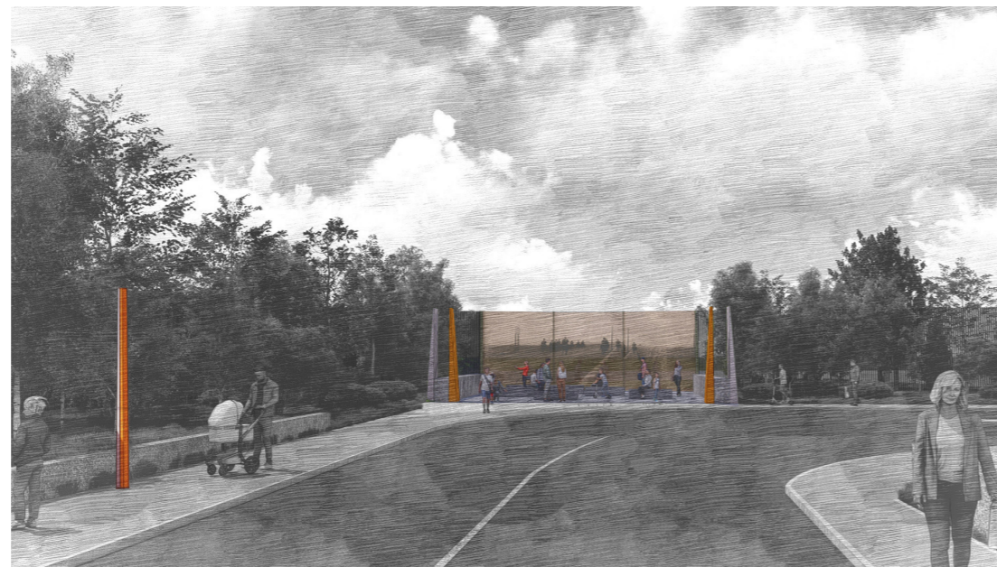
▲ Pigeon House Rd. street view towards proposed 4m high noise barrier with proposed intermediate markers Type C at 30m centres, courtesy of BRIGHT
