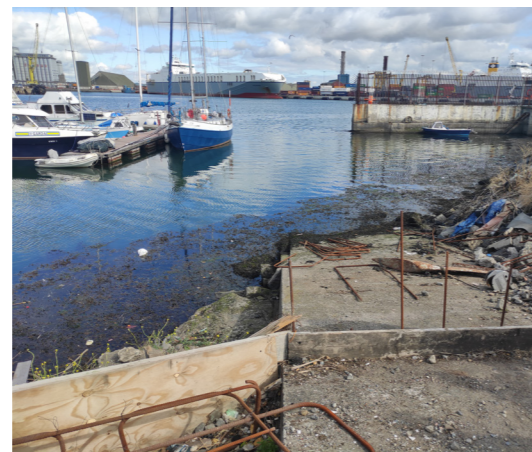
▼ Old redundant slipway to north-eastern corner of site
