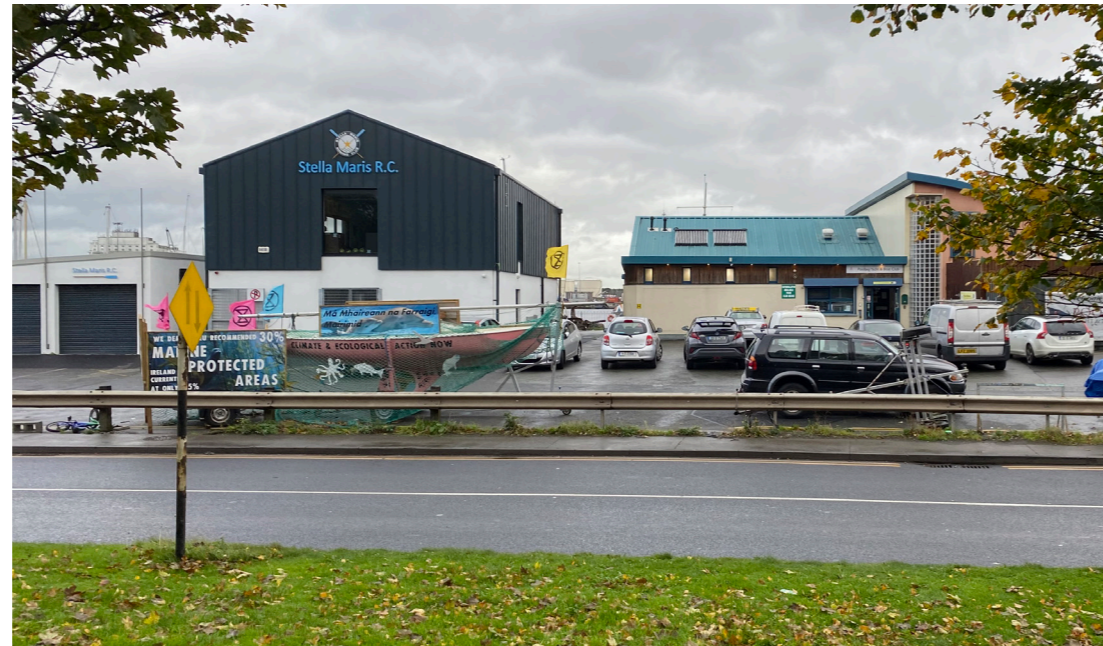
▲ View of existing boat clubs from other side of the East Link Road
