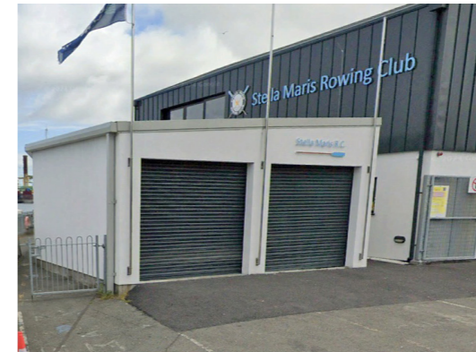
▲ View of existing Rowing Club Store exterior
