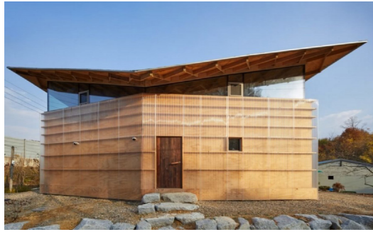
▲ A timber framed assymetric butterfly roof with a generous overhang will continue the expression of the adjacent boat clubs and will provide a counterbalance to the more industrial materials of the shed
