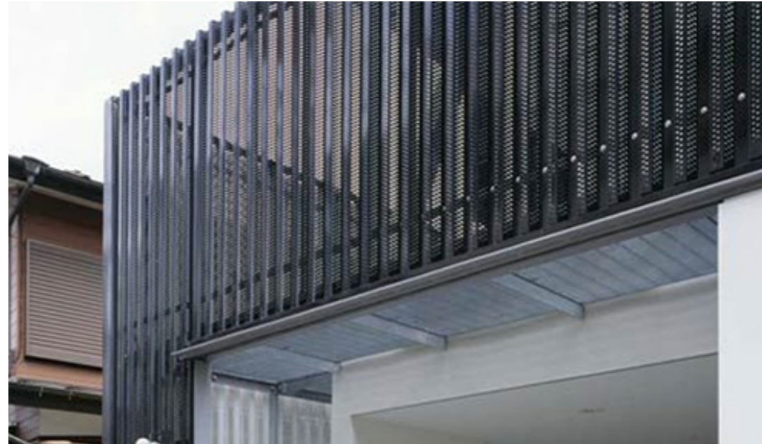
▲ A perforated corrugated metal rainscreen facade will be used to clad the larger elements of the Boat Maintenance Building. This will allow for human scale fenestration to be accommodated behind the facade which will provide interest at ground level and allow a hint of the internal activity to passers by.
