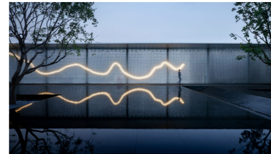
▲ Example of a light installation to building facade, depicting the movement of water
