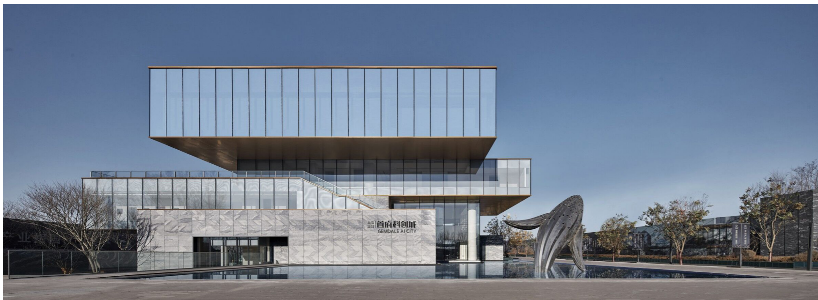
▲ The dramatic cantilevers of the different floors will be most prominent facing the waterside where the stepped volumes are reacting to the internal building programme and the need for maximizing views and connection to the water.
