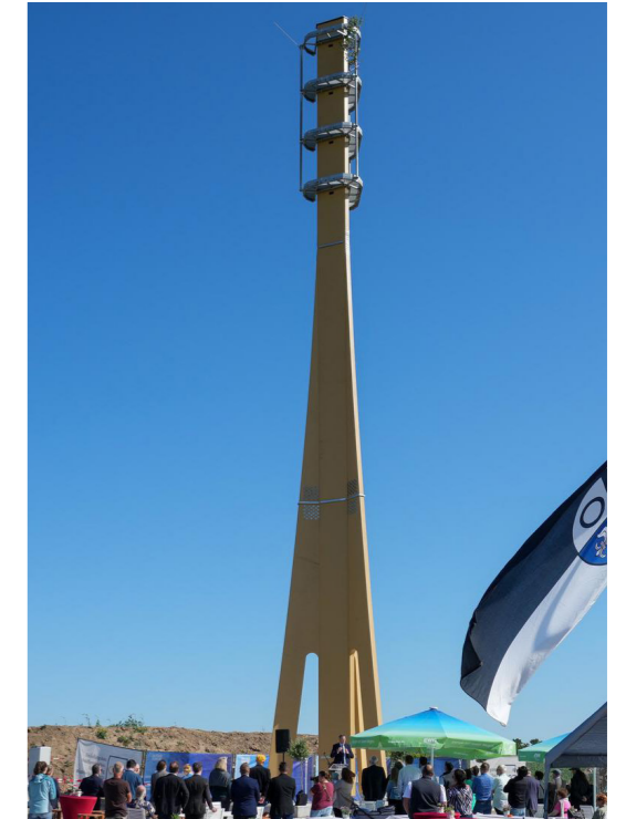
Precedent Image of timber glulam mast structure in Bechtolsheim Germany
