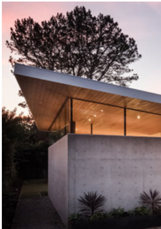
▲ A generous clerestory separates the expressed roof from the more solid plinth elements of the shed, allowing for a clear legibility of both and also ensuring a good level of daylighting to all interior working spaces.
