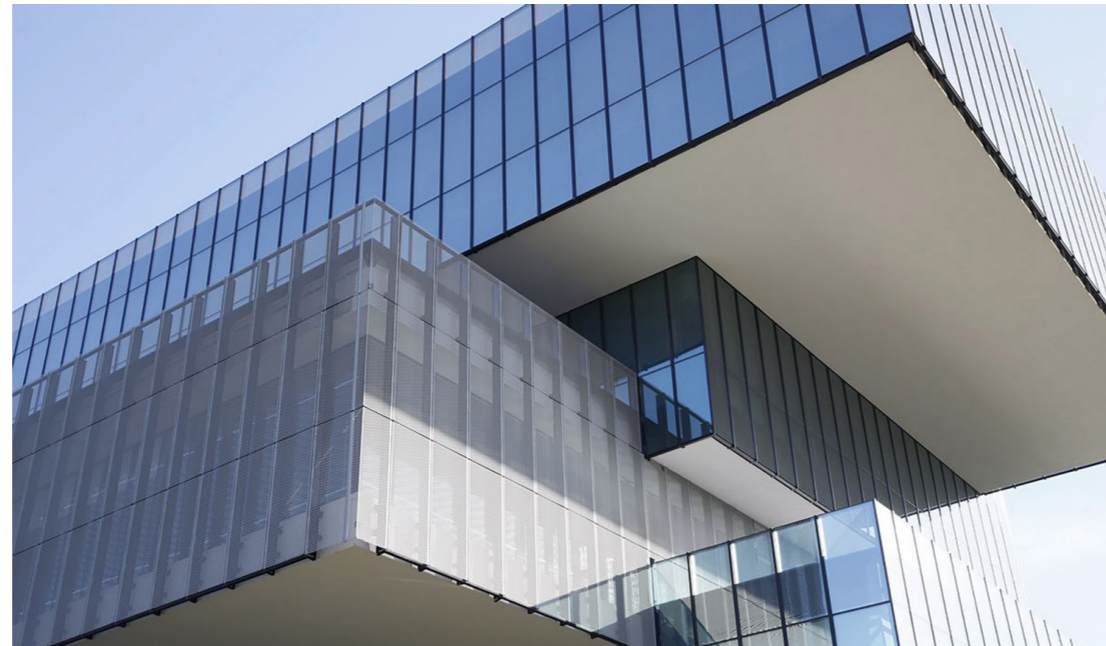
▲ The simplicity of the repetitive grid and flush detailed glazing help to emphasize the clear expression of the sliding volumes
