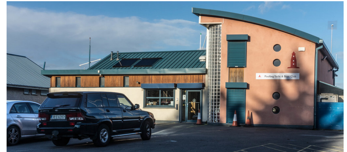
▲ Exterior view of existing Poolbeg Yacht & Boat Club facility
