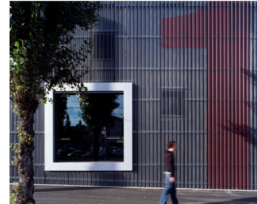
▲ Example of a perforated metal rainscreen facade which provides an appropriate industrial materiality to the building, whilst also allowing for a more playful expression accommodating varying degrees of openness paired with potential signage integration behind facade.
