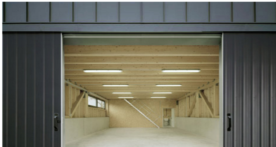
▲ Large scale hangar style sliding doors will be contained within a supporting expressed steel frame and when left open will provide a generous view of the shed interior with its contrasting warm timber interior
