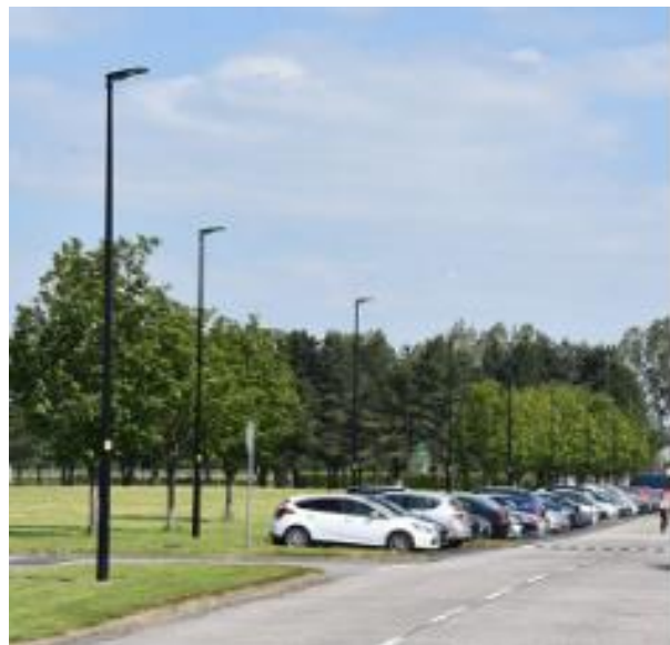
Metro Streetlight - Veelite IP66 IK 09 - 625mm x 290mm x 105mm Location: Maritime Villiage – Boatyard & Harbour Operations Building Carpark
