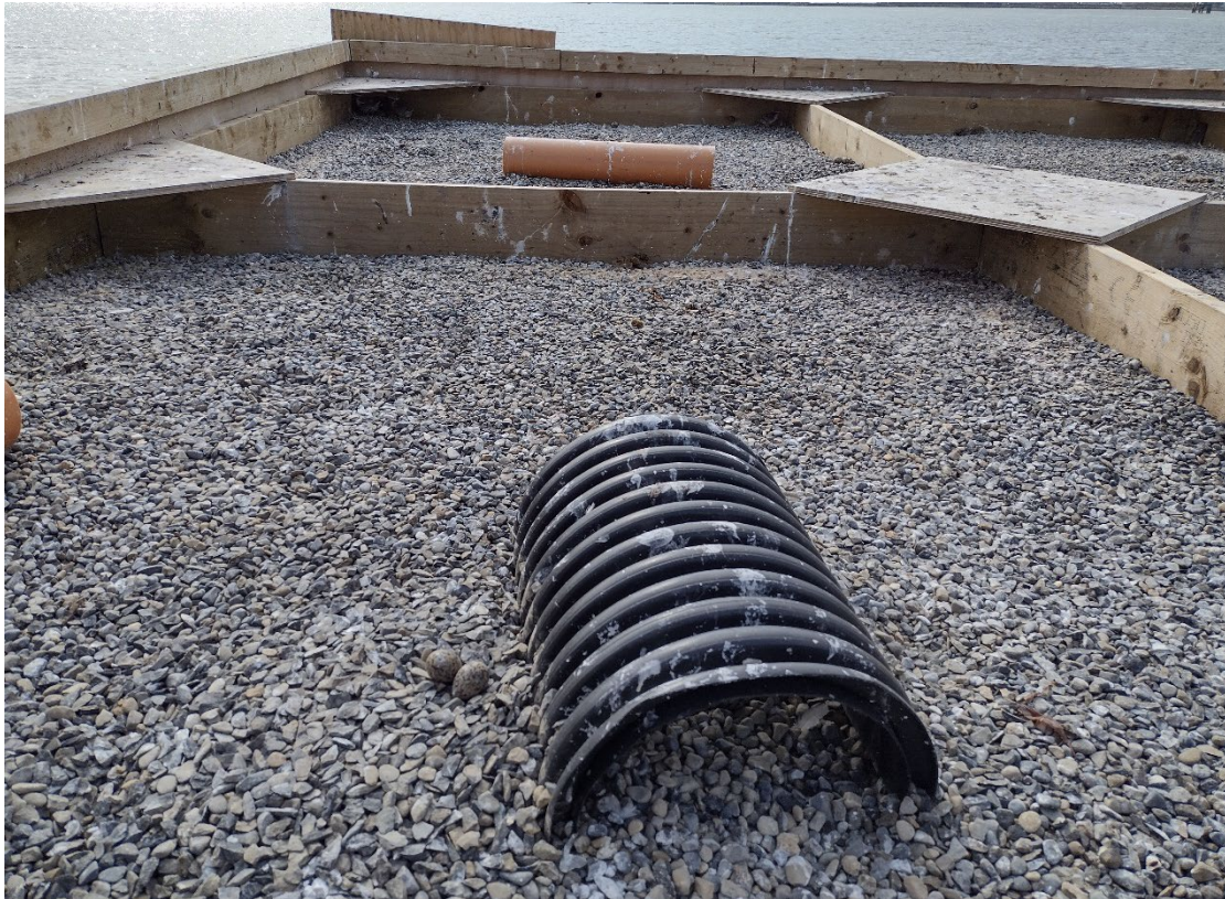
Pipe shelters on tern platform, Dublin Port
