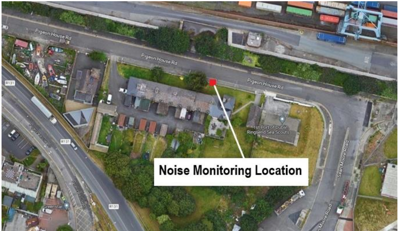
Figure 12.1.4 Coast Guard Cottages Noise Monitoring Location (A-NML1)
