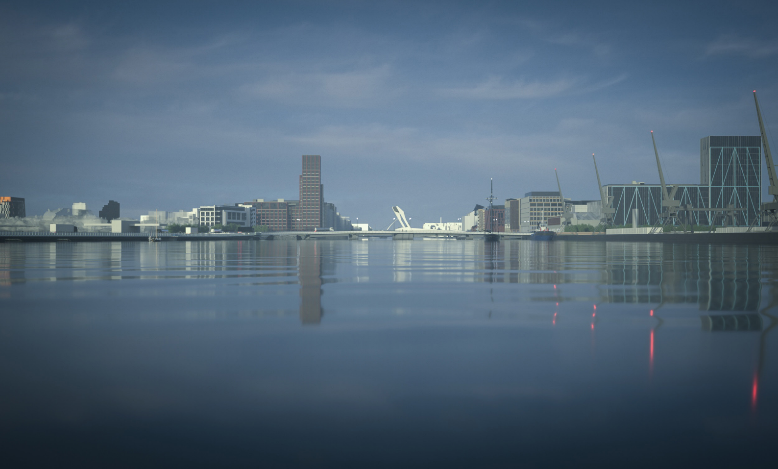
Approaching the SPAR bridge along the navigation channel
