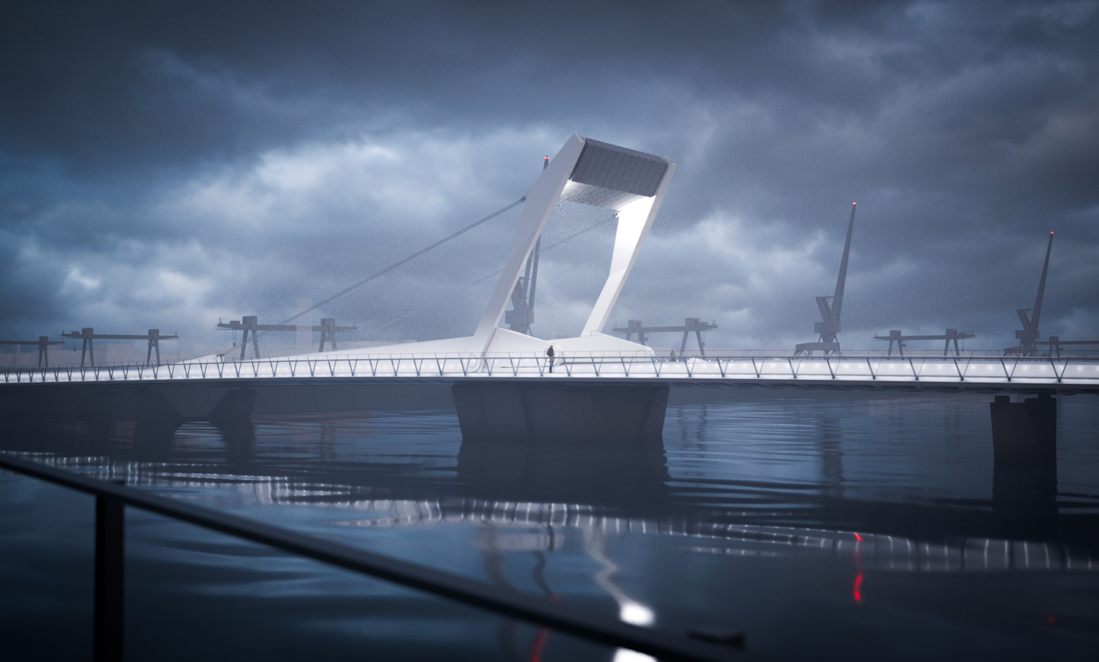
The low level lighting picks out the bridge deck as a ribbon of light
