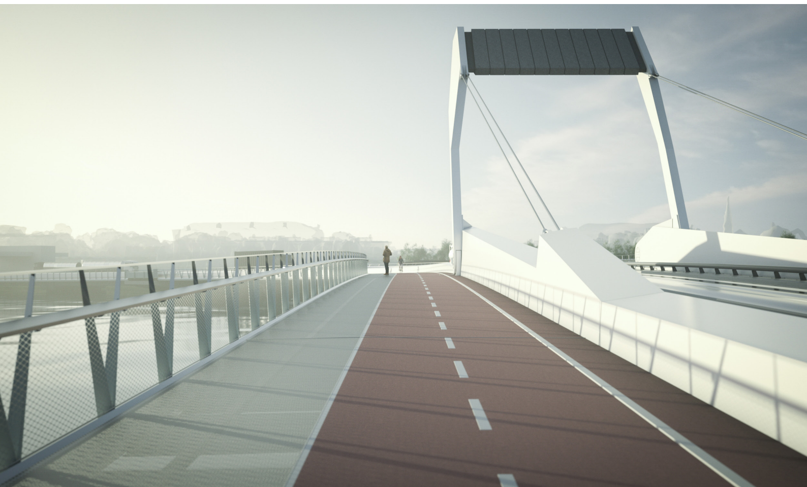
Spine beams at lifting span separate carriageway from active travel walkway
