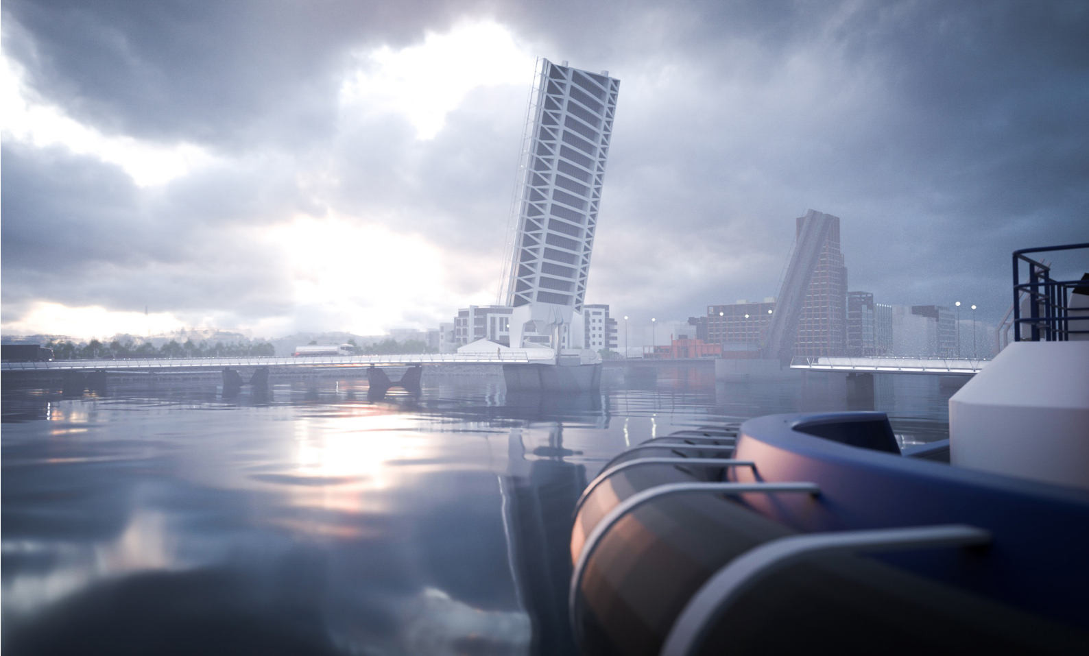
The soffit grid structure is revealed as the opening span is lifted
