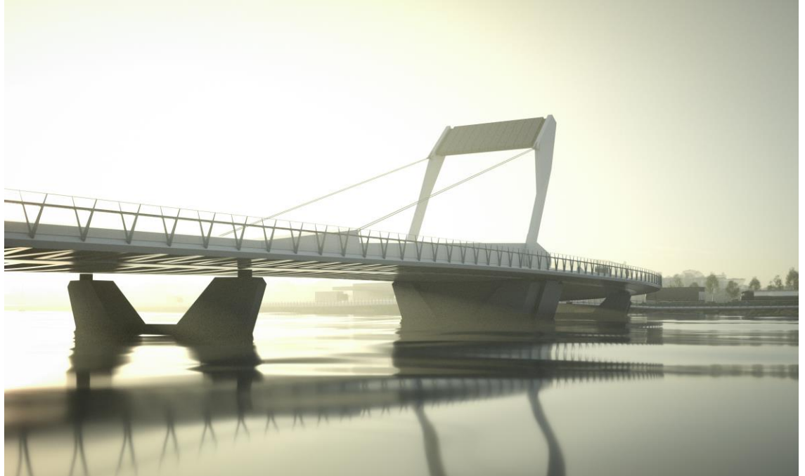
Figure 21: Parapet runs seamlessly across opening spans and approach spans
