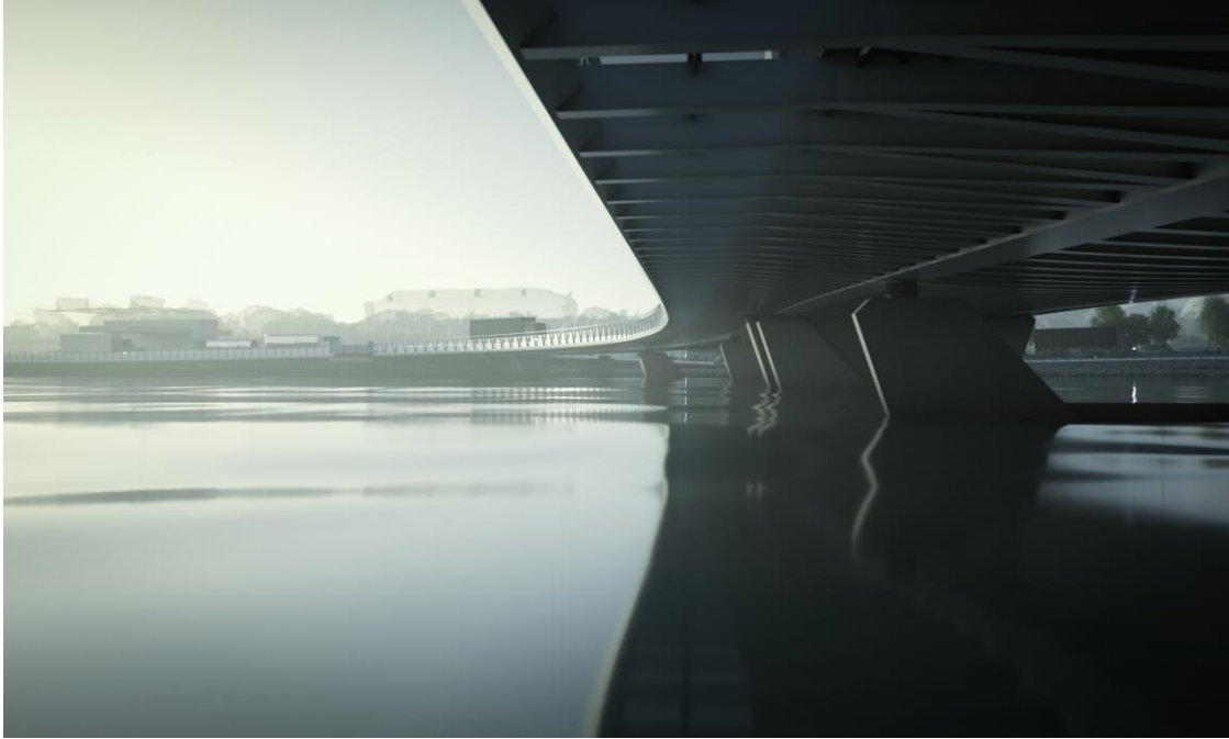
Figure 29: View from river showing SPAR Bridge continuing onto approach viaduct
