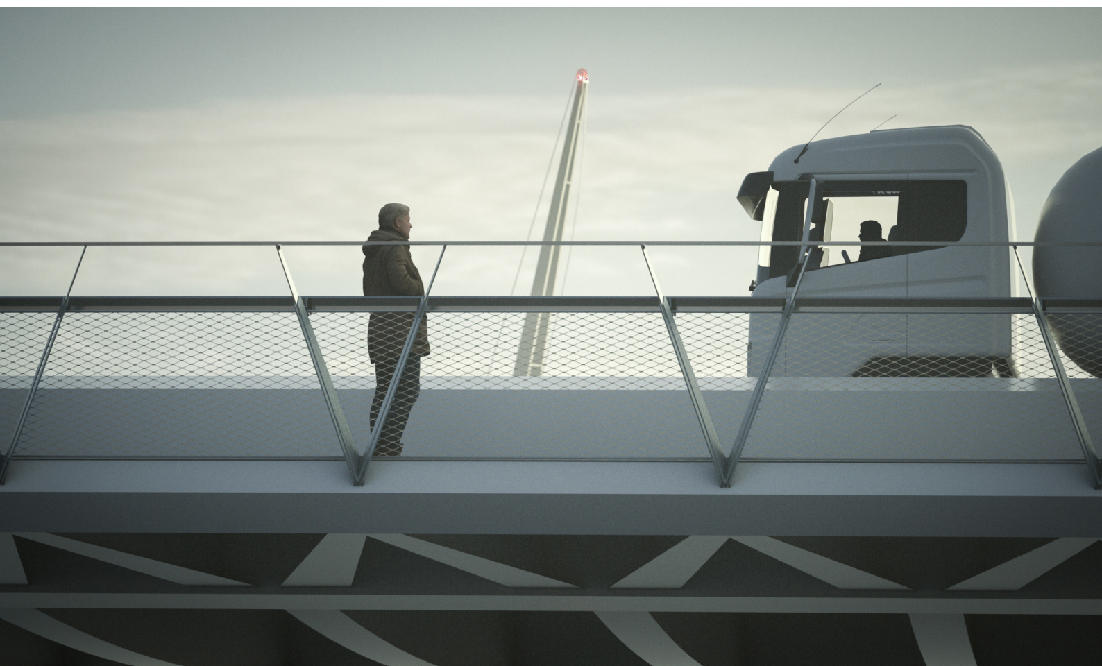
Spine beams separate pedestrians from HGV traffic on carriageway
