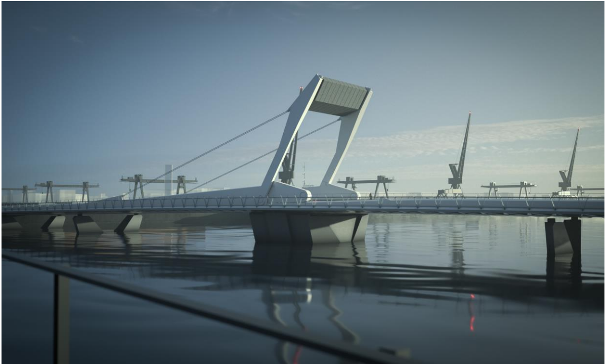
Figure 20: The geometry of the piers allows light to catch the faces differently to break up the visual mass
