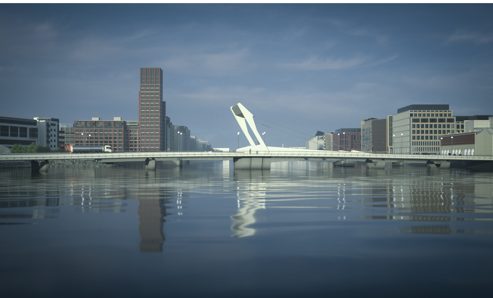
The counterweight gives a distinct identity to the bridge and clearly denotes the opening span
