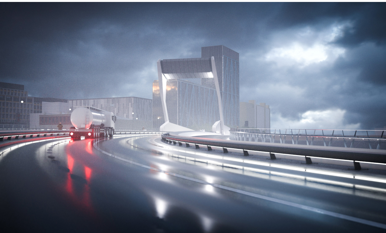
The counterweight provides a gateway element across the road to the port when the bridge is closed
