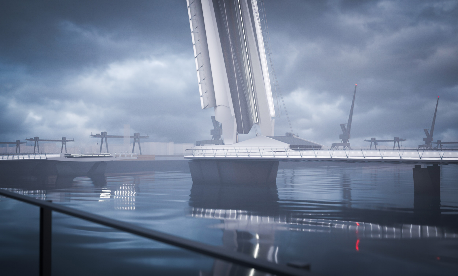
The counterweight aligns with the approach beams when the bridge is open
