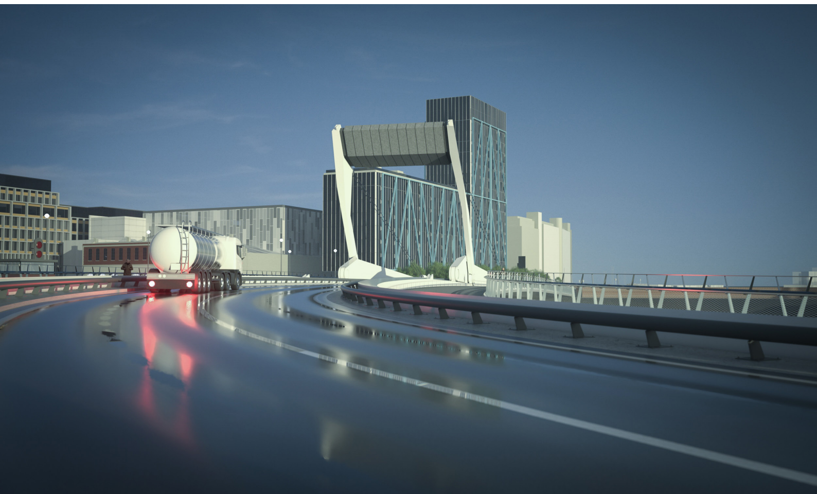
Counterweight forms gateway over carriageway
