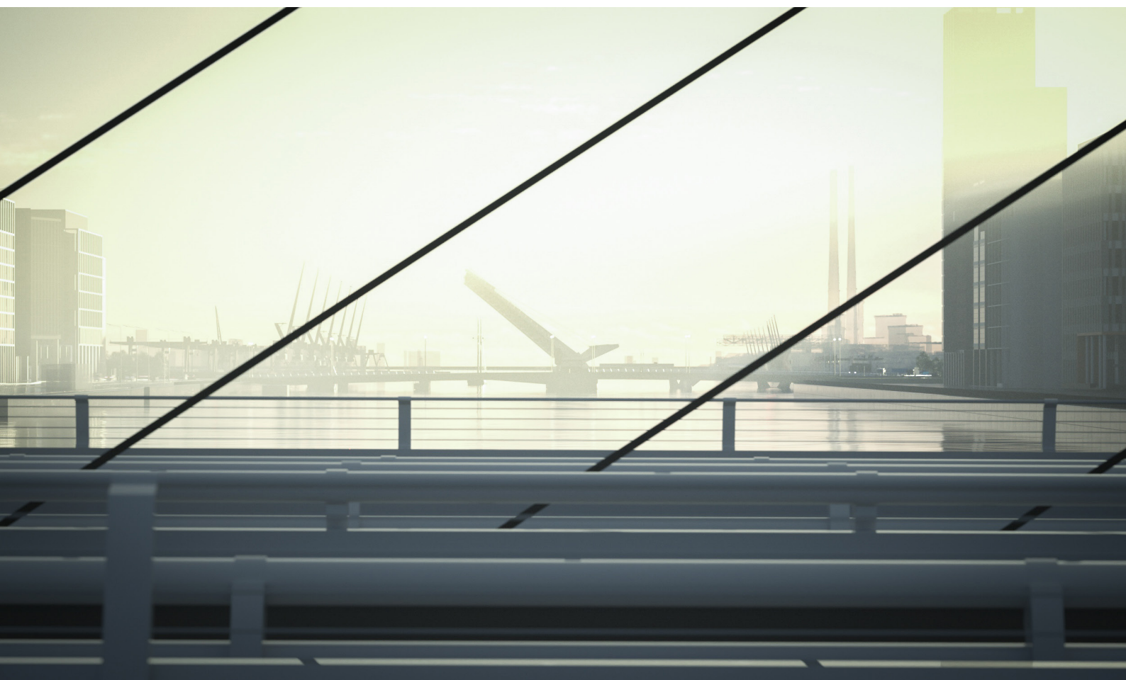
View of SPAR Bridge in a half open position, from the Samuel Beckett Bridge
