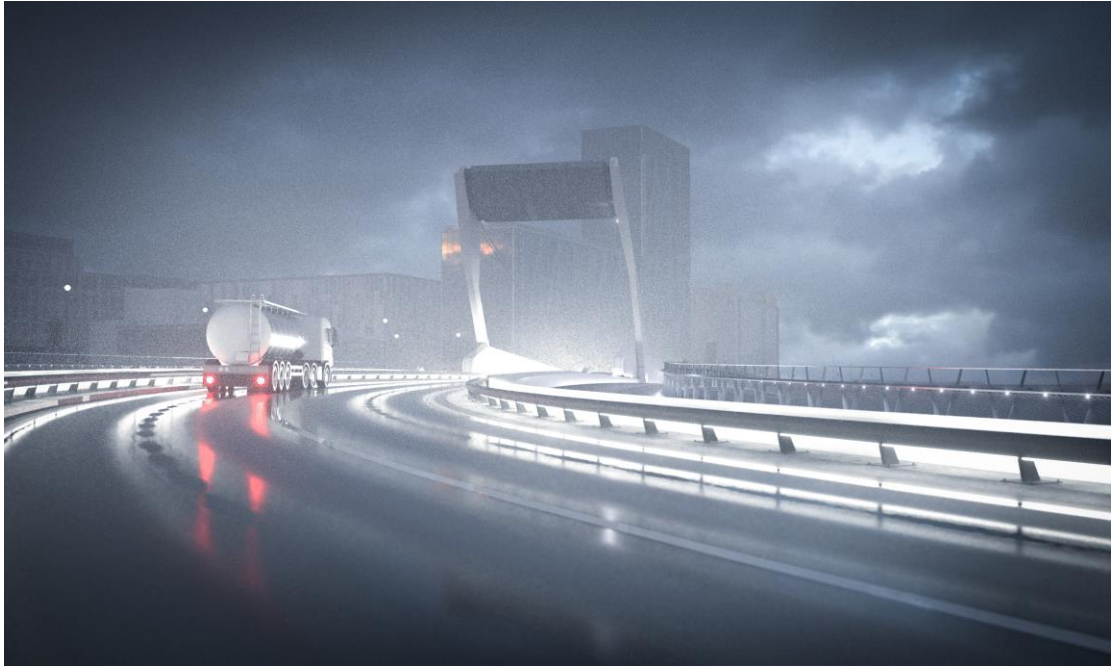
Figure 23: Low level functional lighting on SPAR Bridge
