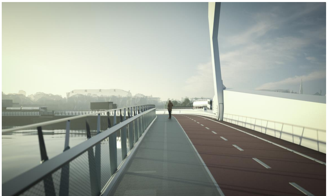
Figure 21: Parapet runs seamlessly across opening spans and approach spans
