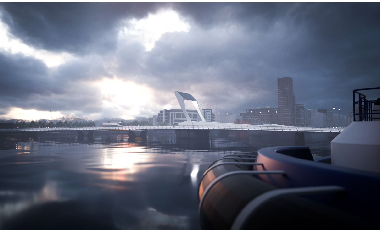
The counterweight provides a distinctive gateway element when the bridge is closed
