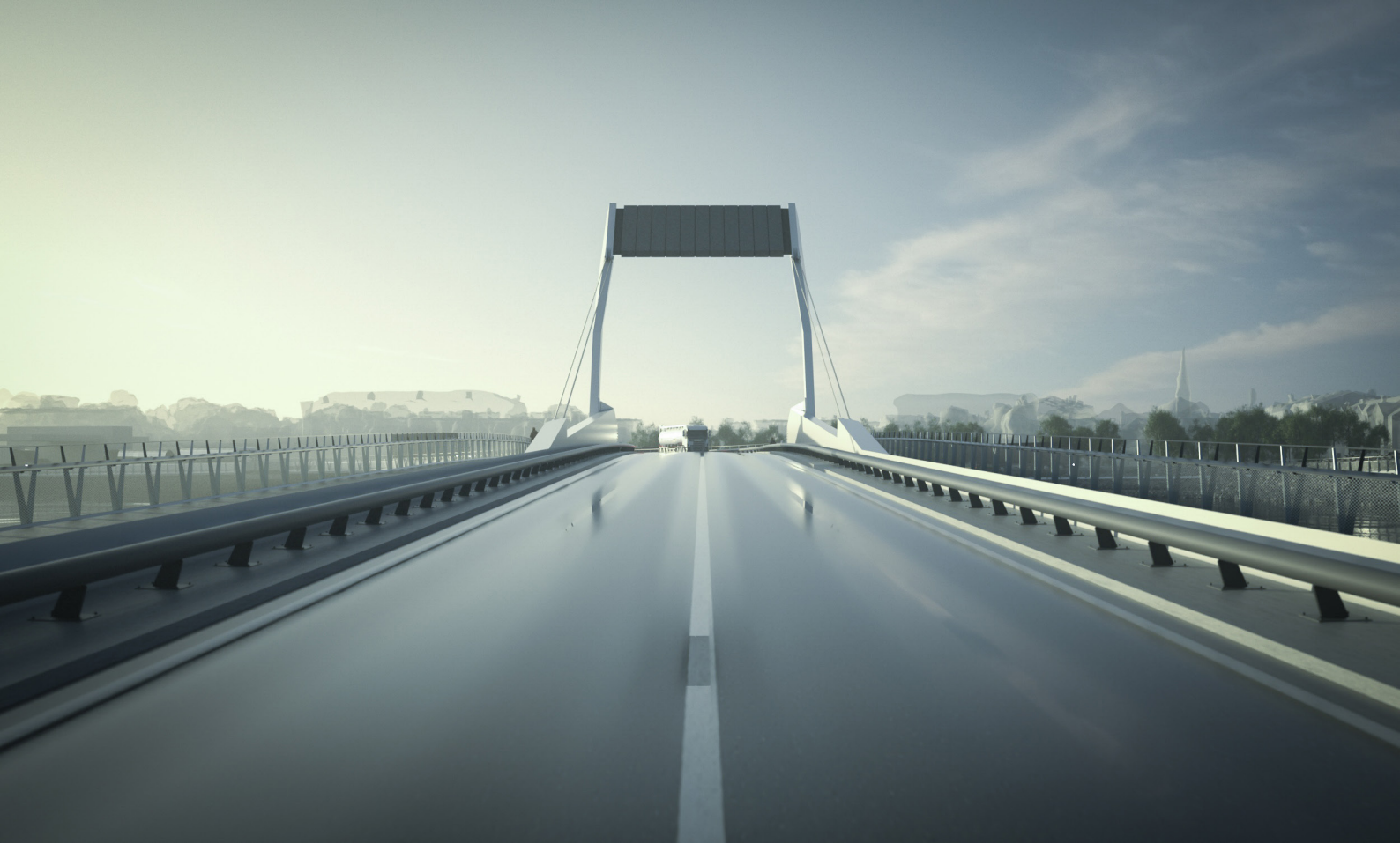
Counterweight forms gateway over carriageway
