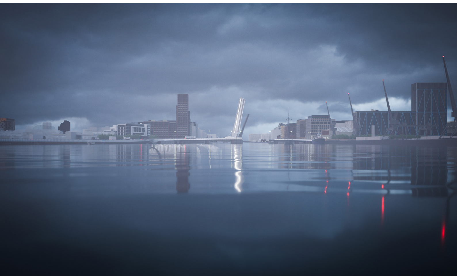
View along the navigation channel from the port side towards the city with the SPAR Bridge open
