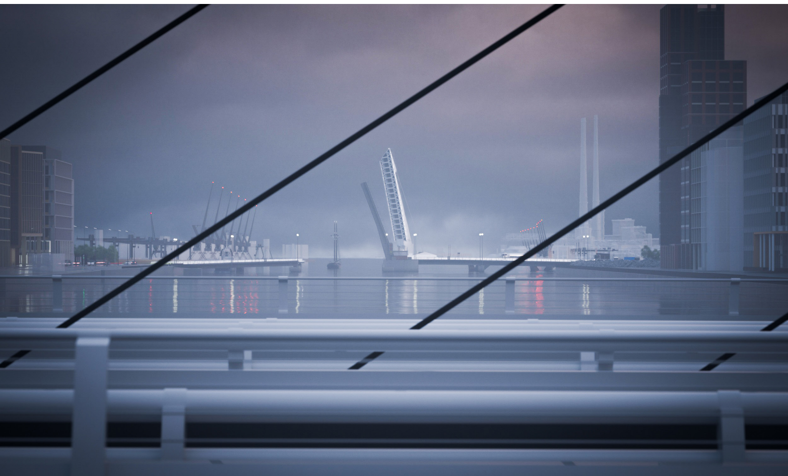
View of SPAR Bridge in a half open position, from the Samuel Beckett Bridge at night
