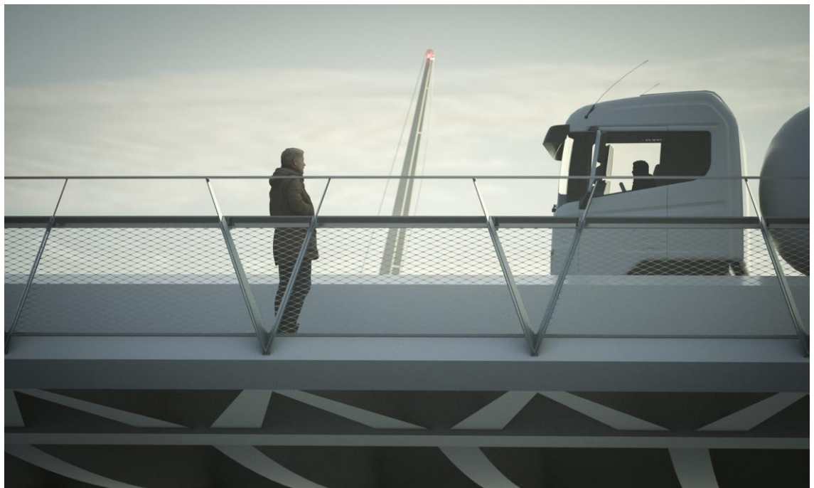
Figure 17: Traffic separated from walkways by spine beams allows a thin, open edge condition
