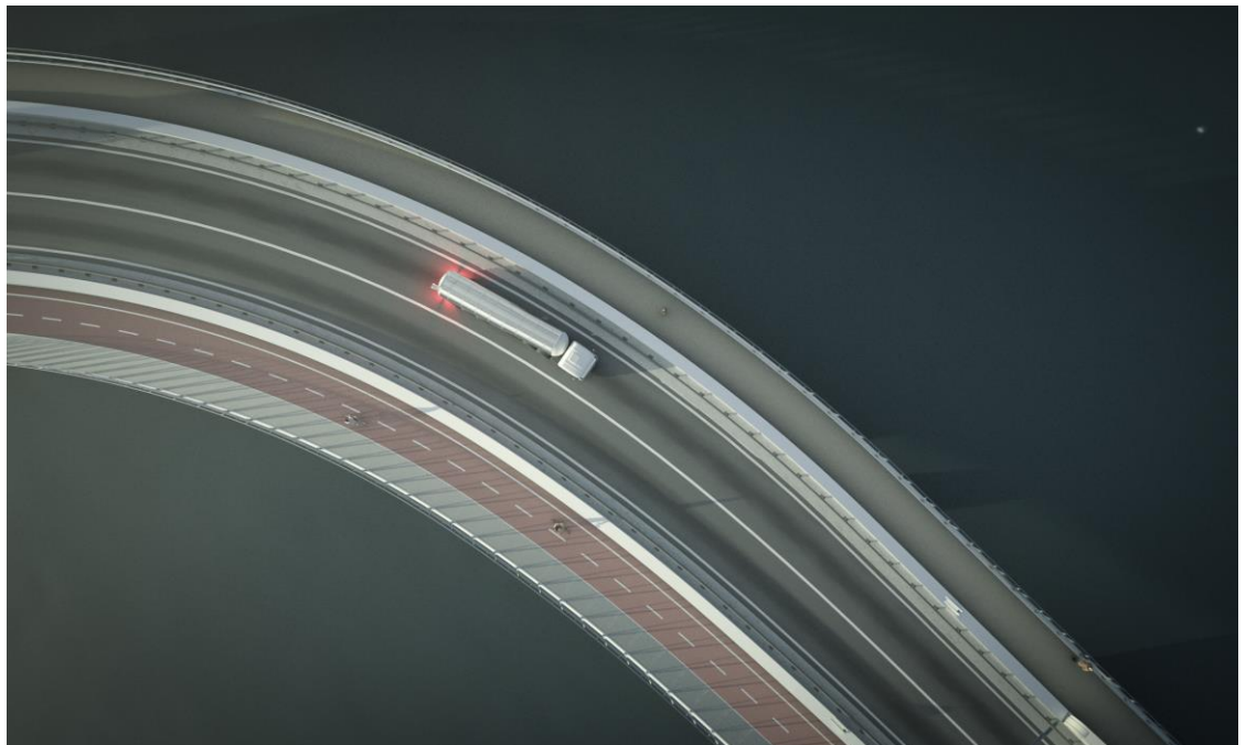
Figure 26: Overview showing changes in surfacing across deck.
