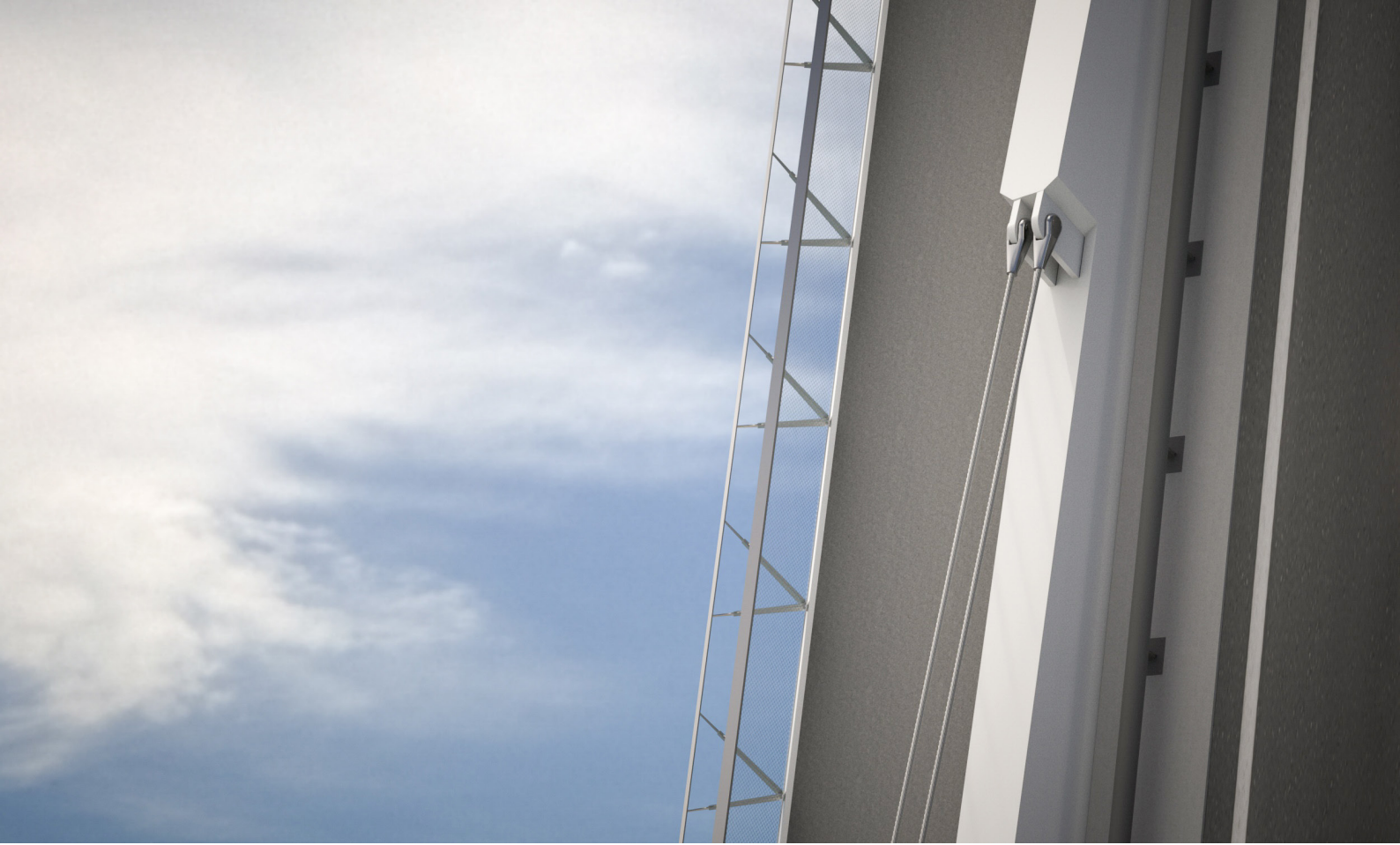
Tip of spine beams shaped to accept cable connections
